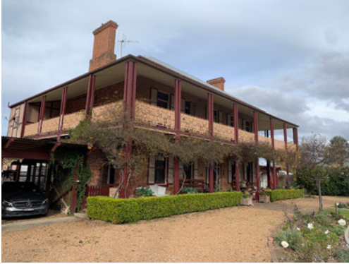
Figure 3: Western (front) and northern elevations, as viewed from the front garden.
