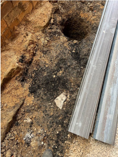
Figure 24: Evidence of the location of a former kitchen oven or stove found under the later addition brick paving to the southern verandah at ground floor level.
