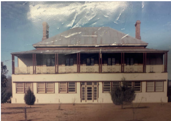
Figure 23: Bleak House while in use as flats in the mid to late 20th century. Courtesy of the Mudgee Museum.
