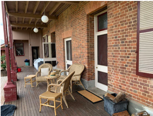
Figure 7: Eastern ground floor verandah with enclosure at south-eastern corner.
