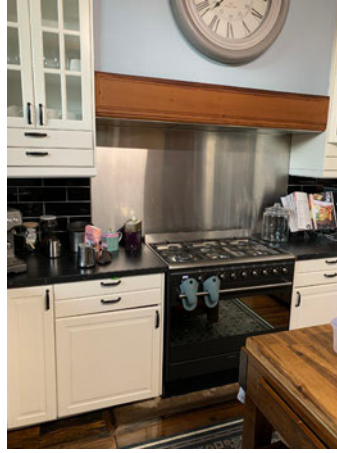
Figure 13: Original chimney breast partially removed by previous owners to accommodate stove. A new door opening is proposed in this location.
