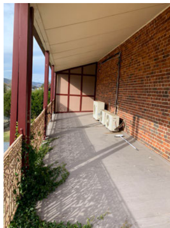
Figure 10: Enclosure at south-western corner at first floor level.
