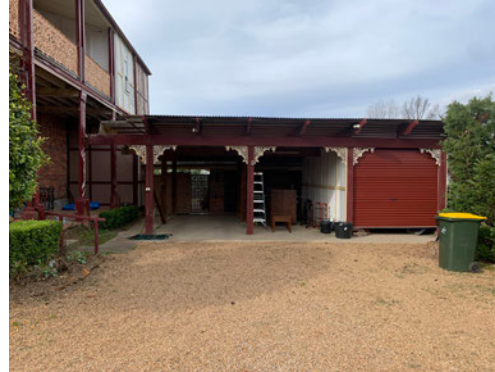
Figure 6: The southern carport with garage.
