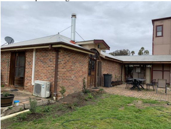
Figure 7: Existing secondary dwelling, to the southeast of the main house.
