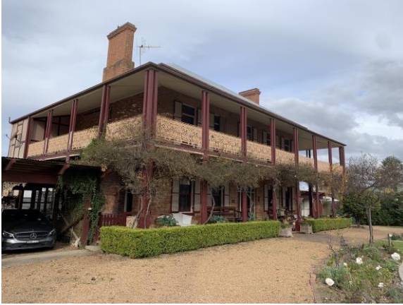
Figure 3: Western and northern elevations, as viewed from the front garden.
