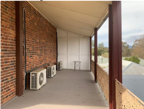
Figure 5: Southern verandah, looking east towards existing infill. The proposed walk-in robe and ensuite are proposed to be contained within the existing verandah space along this elevation.
