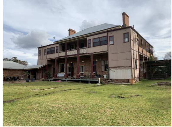
Figure 4: Eastern and southern elevations, as viewed from the rear garden.
