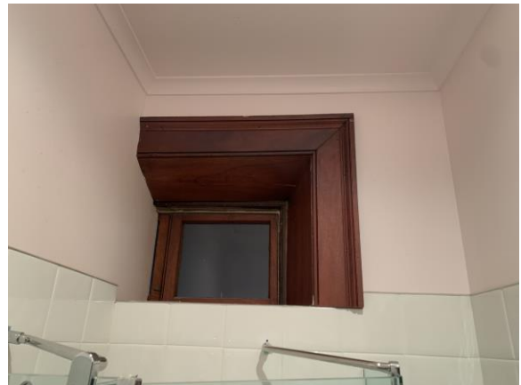
Figure 8: Original window in bathroom to be restored.
