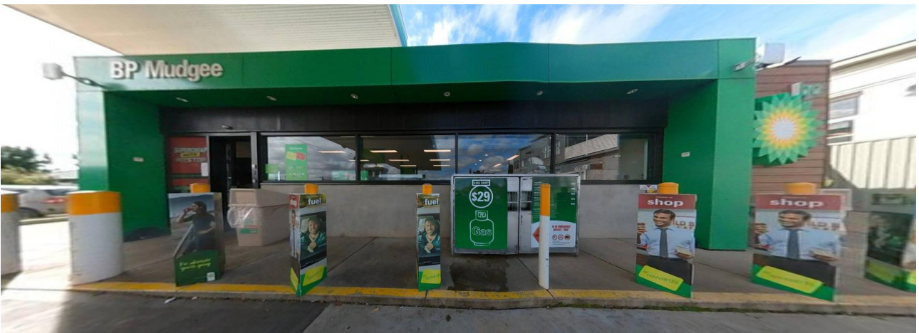
Figure 3: View of existing front facade (source: TFA Project Group)
