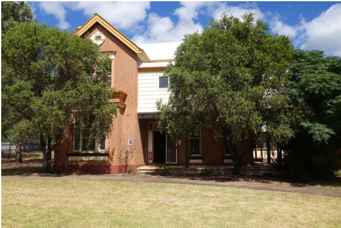
Figure 1 Front View 70 Court Street Mudgee 3 rd February 2021. BH.
