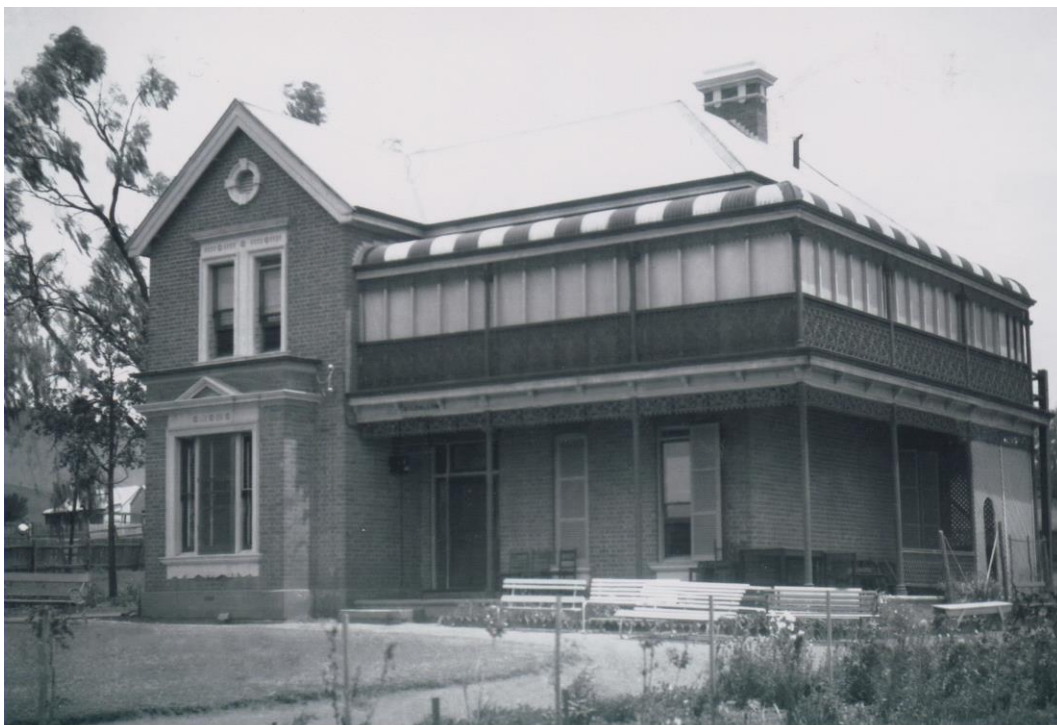
Figure 6 Historic Kildallon image 2 courtesy the Mudgee Museum. Note verandah and landscape details. This image of unknown date probably relates to the 1945-50 period when the CWA opened a hostel for girls. The verandah had been enclosed but the original fabric is still extant.
