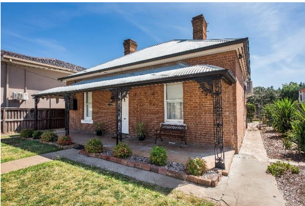
Figure 9: Reverse curve roof of a listed house at 58 Denison St Mudgee. Image by Amber Hooper.
