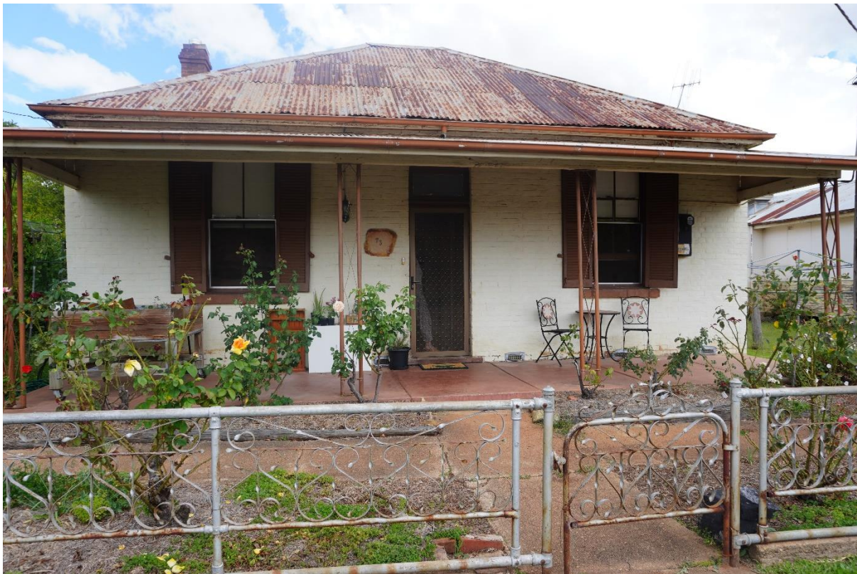
Figure 1 front elevation. BjH March 2022, illustrating the existing verandah replaced in the mid-20 th C . Image 4 th March 22
