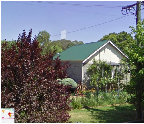
10 LAWSON STREET – BEFORE ADDITION
