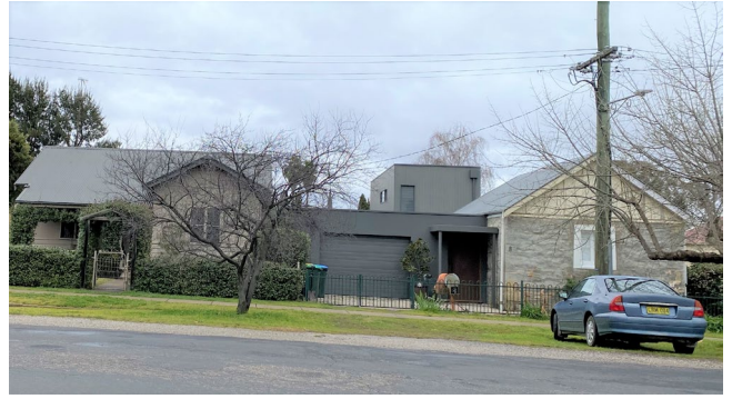
10 LAWSON STREET – AFTER ADDITION
