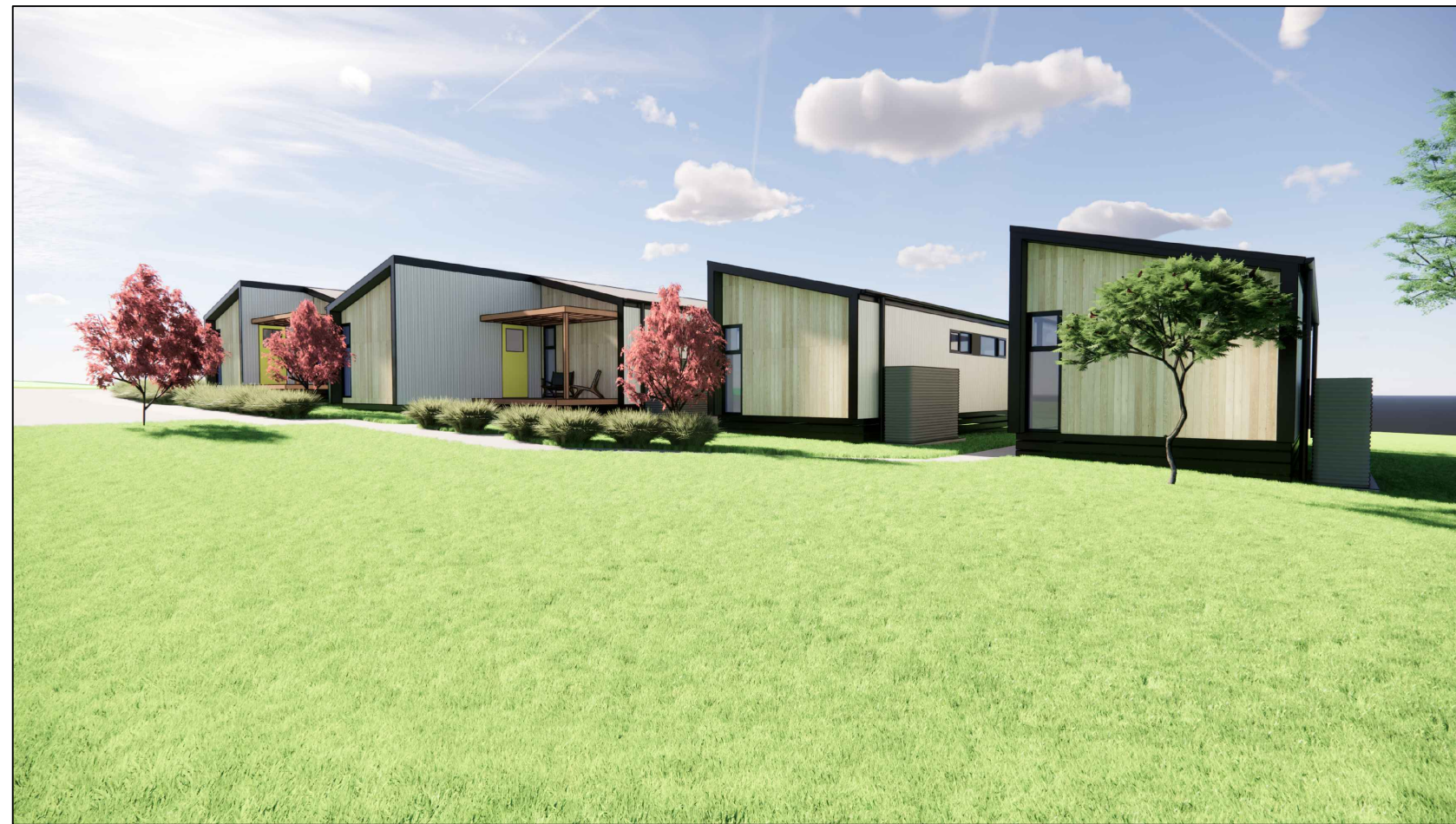
VIEW FROM NORTH EAST
