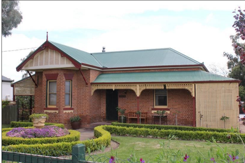
Figure 9: 44 Horatio Street, a heritage item to the south west of the subject site.
