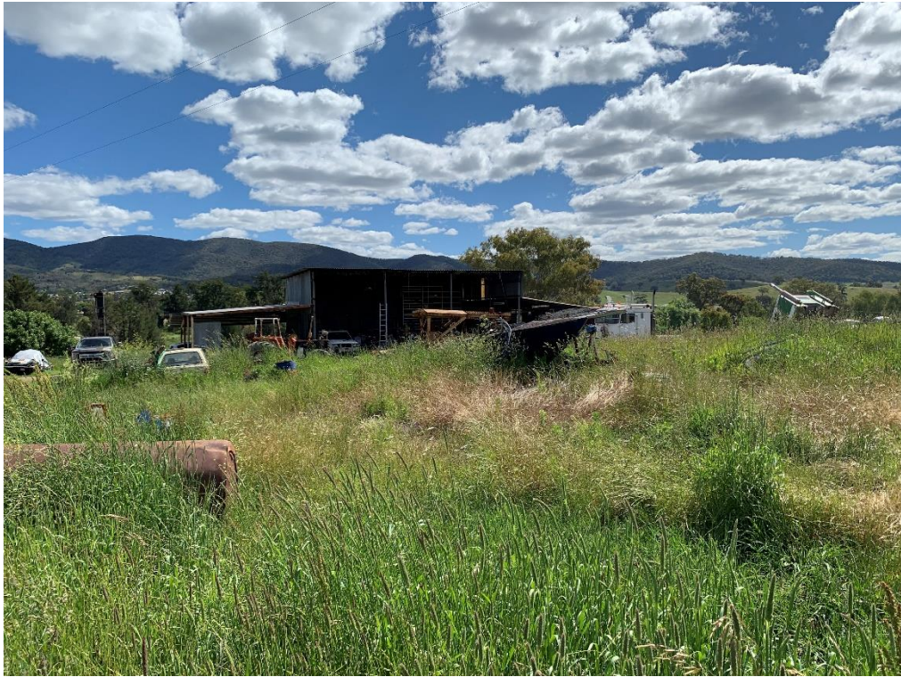
Plate 3 – General view of proposed building B location facing south.
