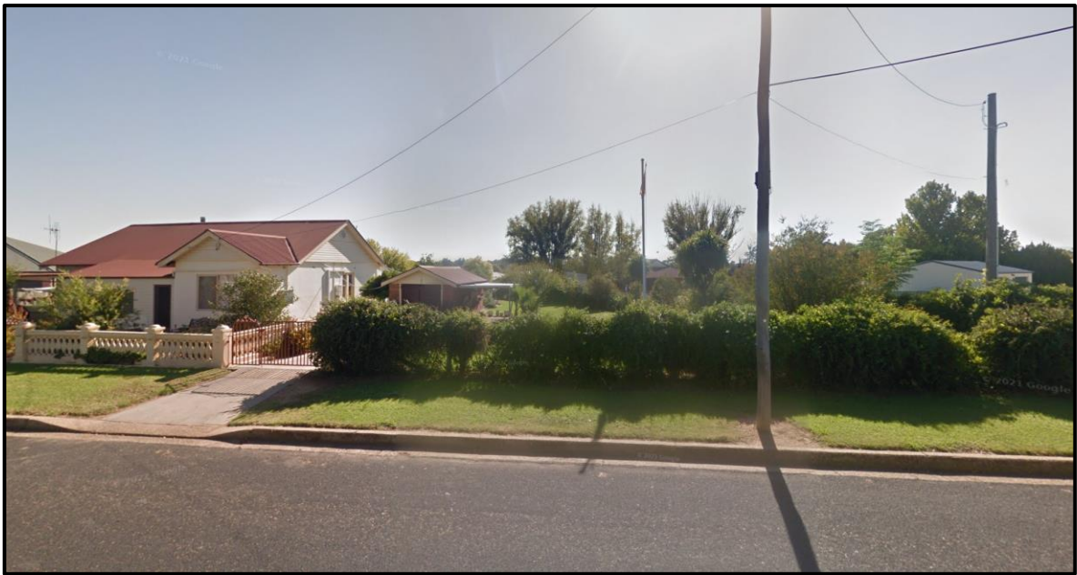
Figure 4: Street view image of the immediate western neighbour at no. 234 Mortimer Street, Mudgee
