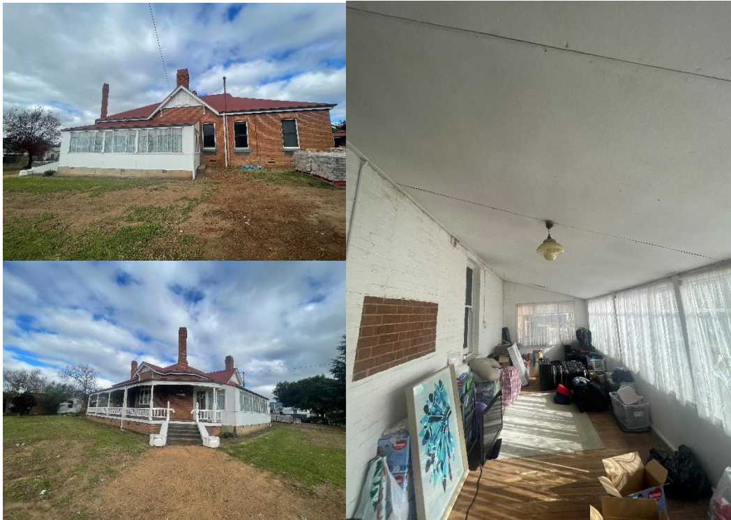
Figure 2 : Photos of the Non-Original Enclosure proposed to be demolishing
