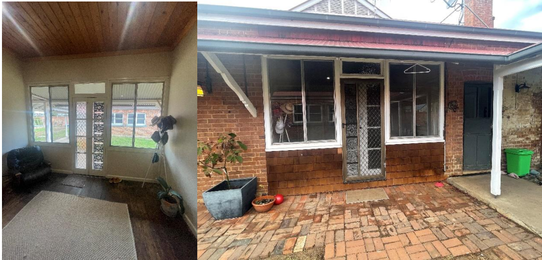
Figure 4: The Aluminium windows and rear double door proposed to be demolished
