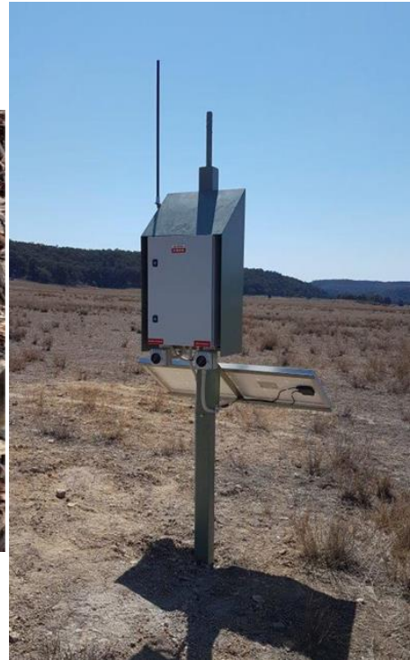
Photo 3.1 and 3.2 Typical Bubble Pot Sensor and Instrumentation Cabinet
