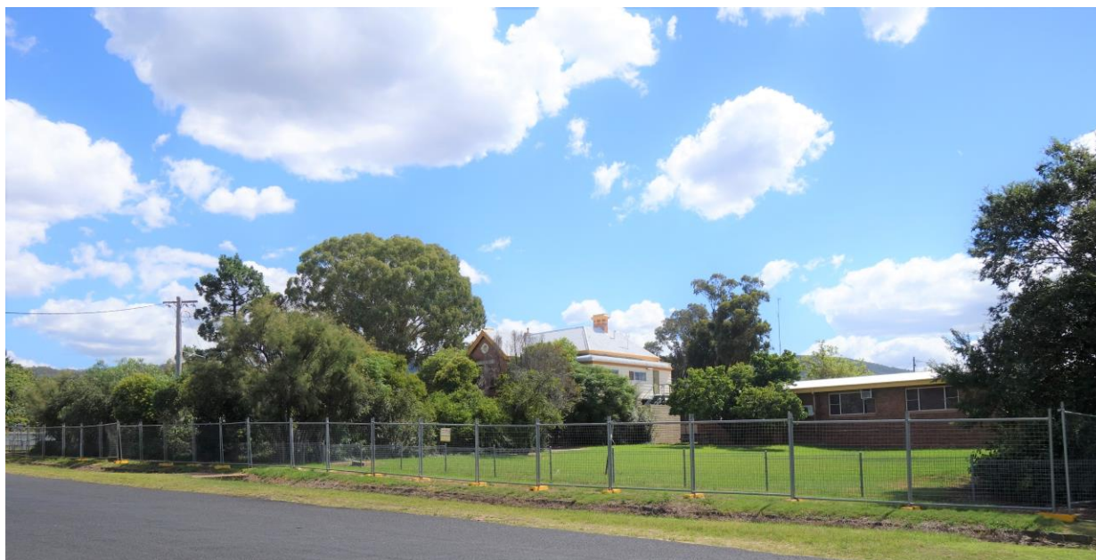
Figure 3 Existing street view of 70 Court Street Mudgee.
