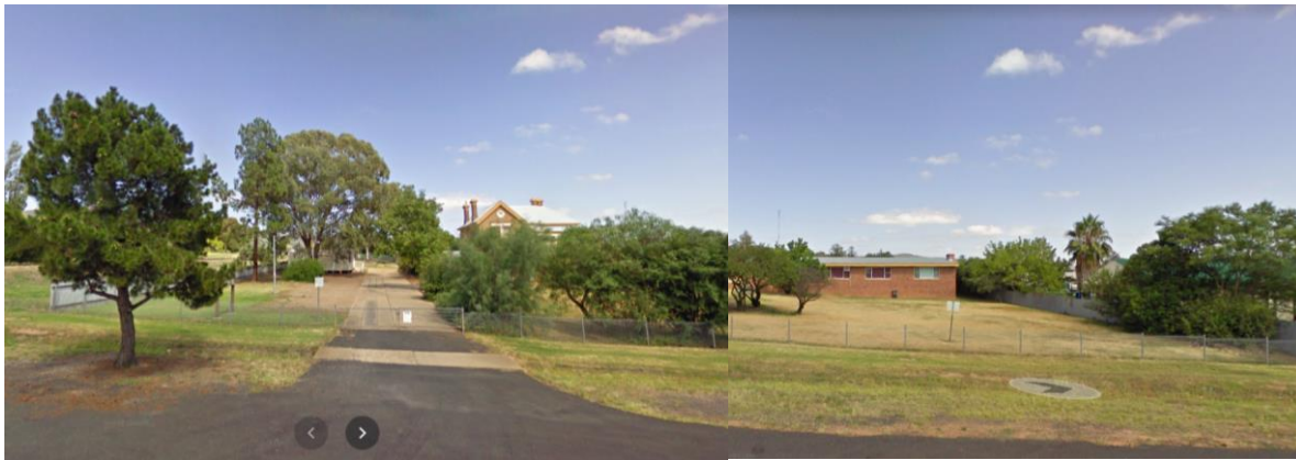
Figure 7: Google Street maps images above show that, although set well back, the dissimilar development of c. 1960s plain brick classroom wing dominates the site. The TAFE wings are not hidden by landscaping, as the Kellett house is. The landscape effect needs to be reversed.
