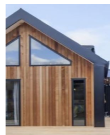
EXTERIOR CLADDING - NORTHERN & SOUTHERN WALLS - JAMES HARDIE AXON GROOVED WOOD GRAIN TEXTURE- TIMBER STAINED FINISH
