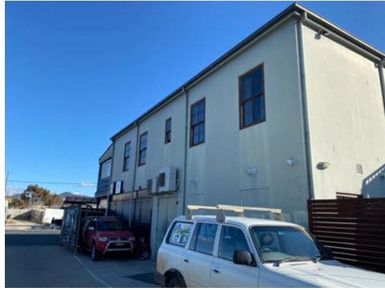
Figure 9: View of eastern elevation facing southwest.
