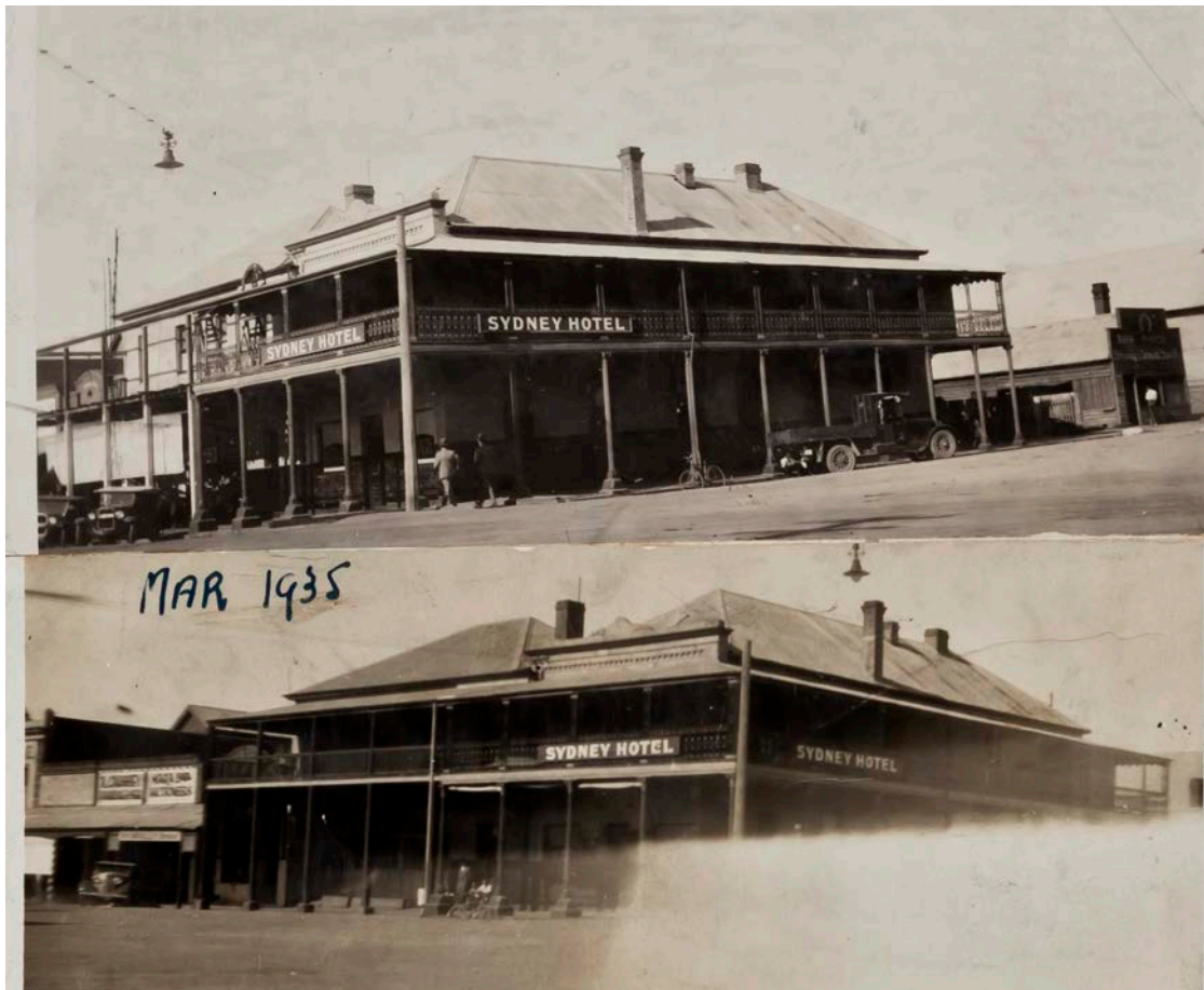
Figure 29: Photograph of the Sydney Hotel during construction (top) of the additions (March 1930) and the completed (bottom) additions (March 1935).
