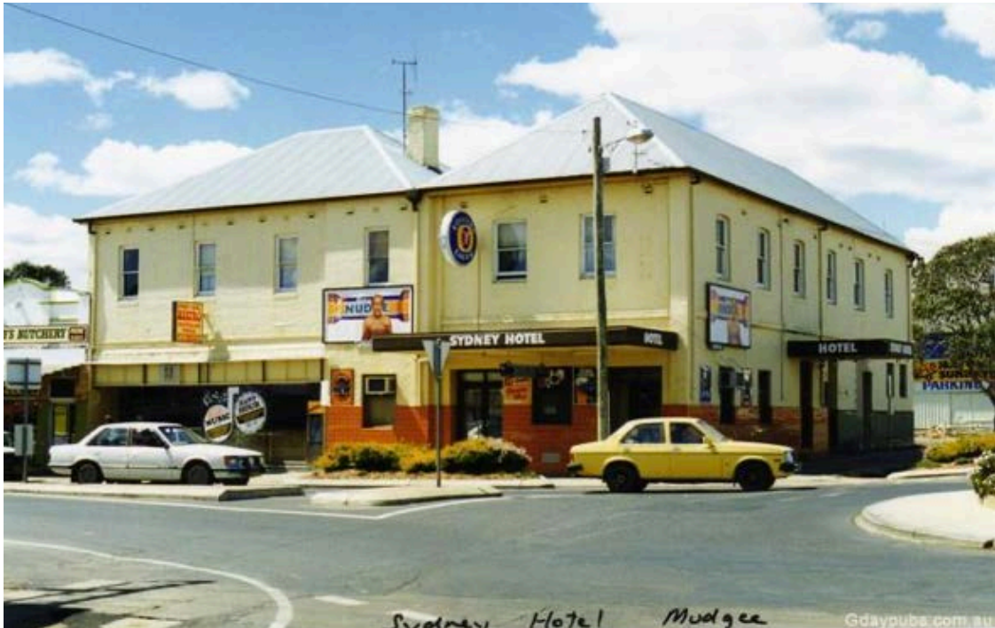
Figure 36: Photograph of the subject site, c.1994.
