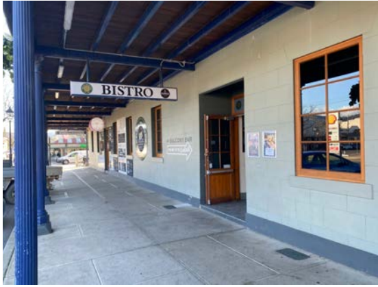
Figure 8: Detailed view of covered footpath facing northwest.
