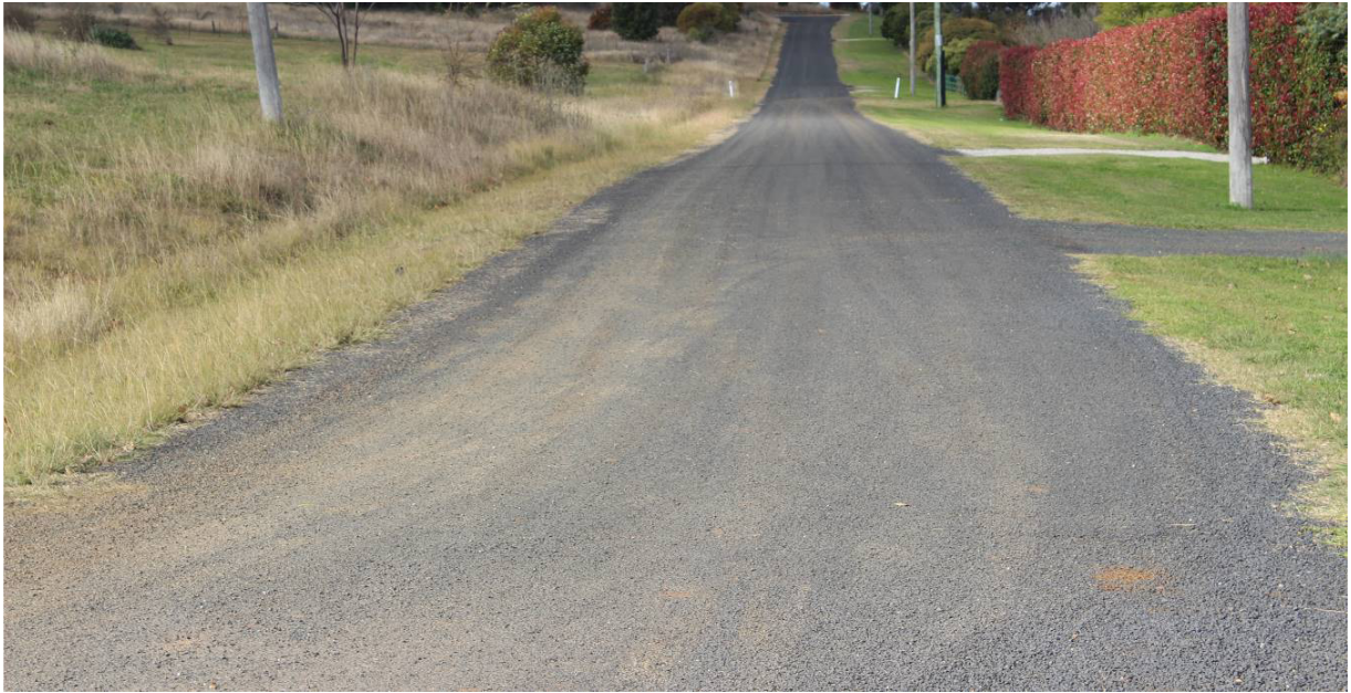
Photograph 5 – Well maintained grassed verge (footpath) on Flirtation Hill Lane
