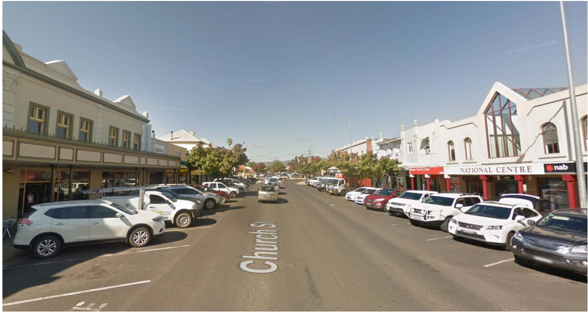
Photo 5 – View southward along Church Street
