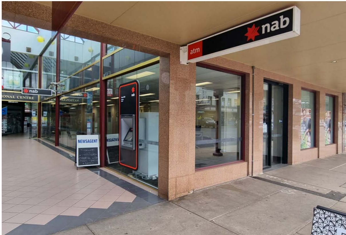
Photo 3 – Corner of Shopfront and Arcade Frontage
