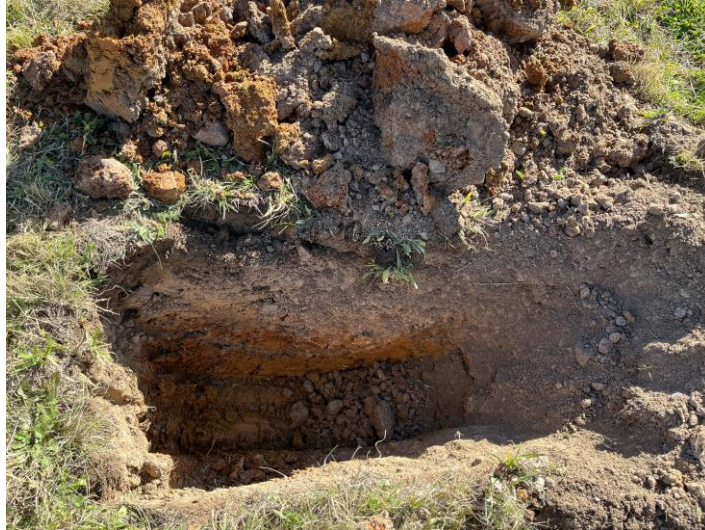
Image 1: Subsoil investigation at the proposed development site
