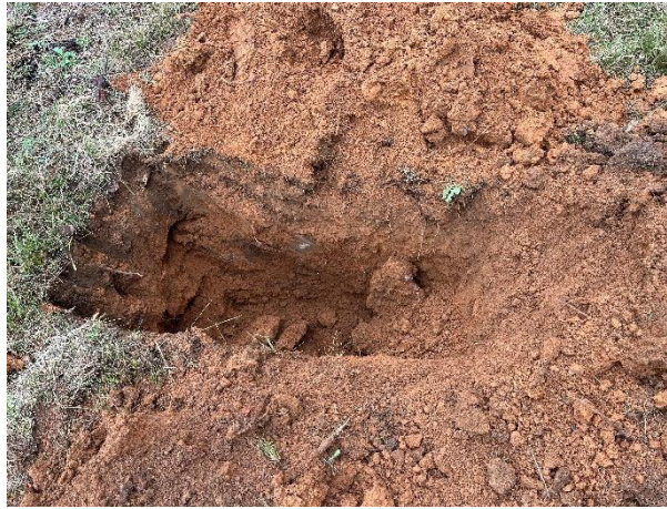
Image 2: Subsoil investigation at the proposed development site 3
