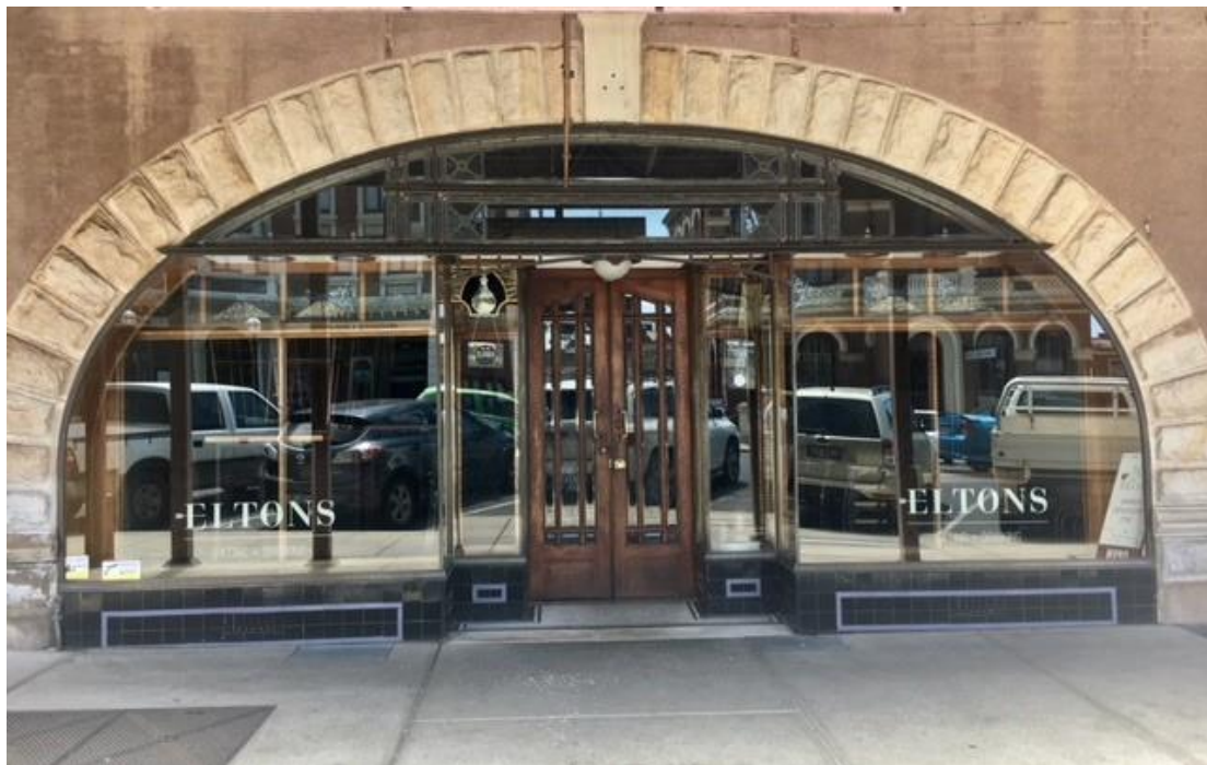
FIGURE 3 FRONT FAÇADE OF ELTONS RESTAURANT
