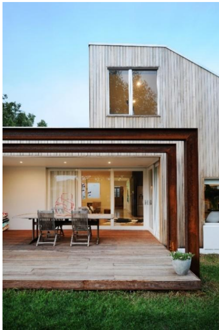
Figure 03 - Existing condition - Rear View
