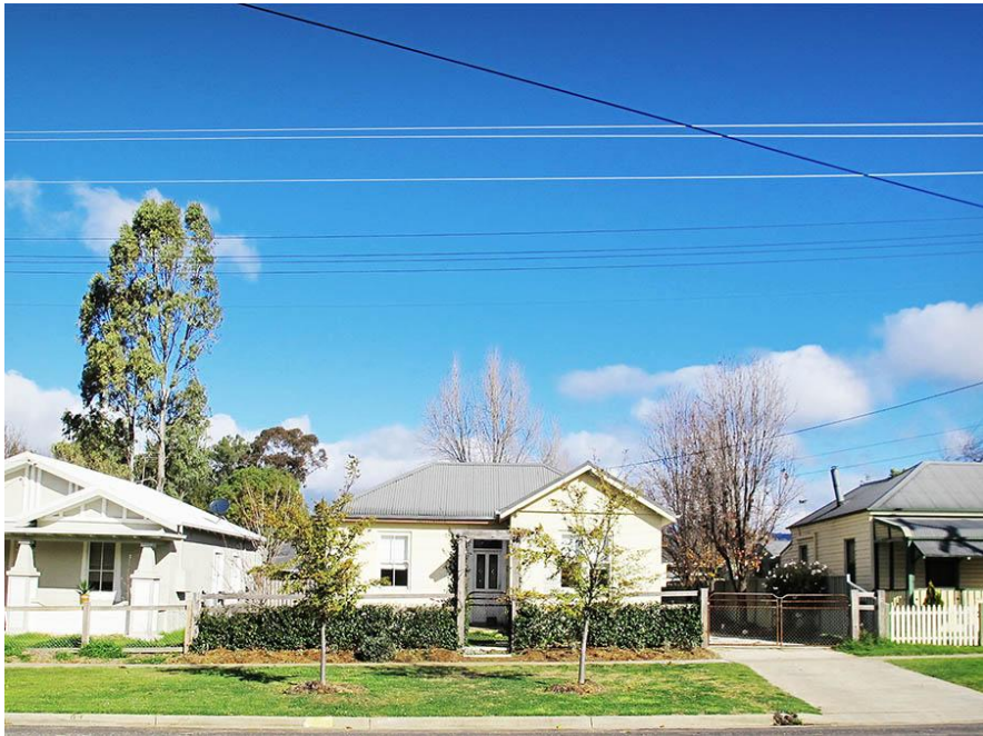
Figure 02 - Existing condition - Front Façade
