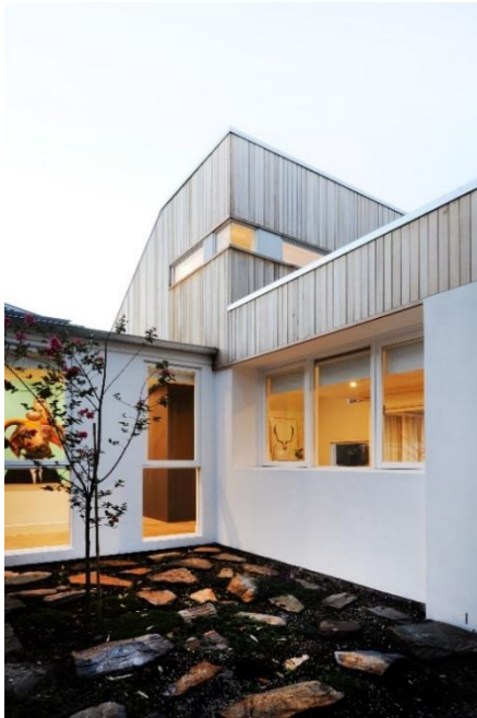
Figure 03 - Existing condition - Courtyard View
