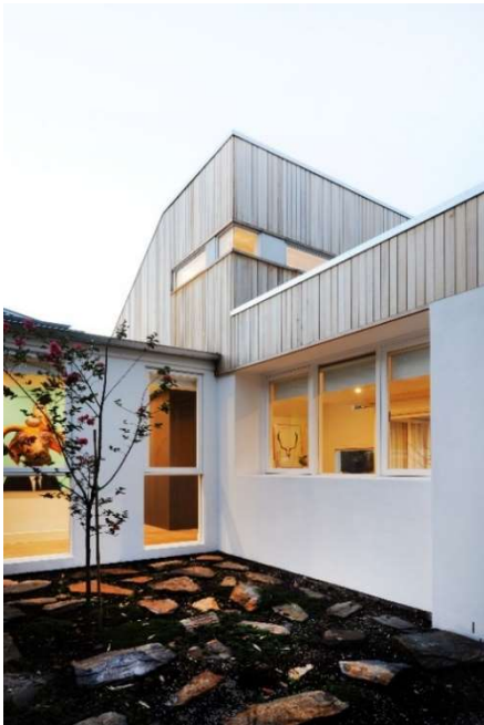
Figure 03 – Existing condition – Courtyard View
