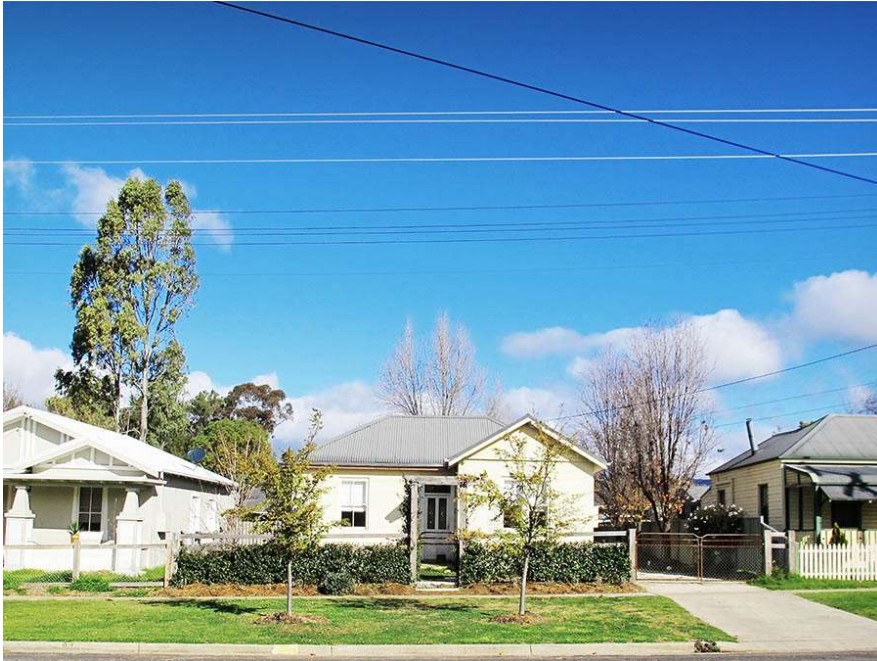
Figure 02 – Existing condition – Front Façade
