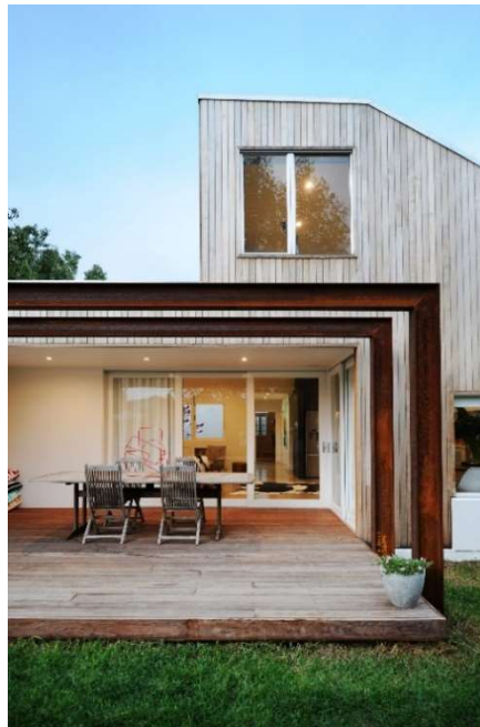
Figure 03 – Existing condition – Rear View
