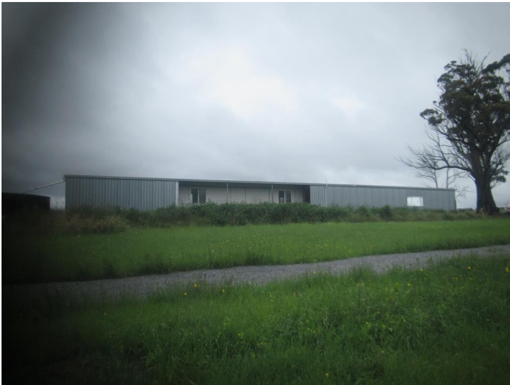
Plate 1 – View of the existing shed subject to alterations and additions
