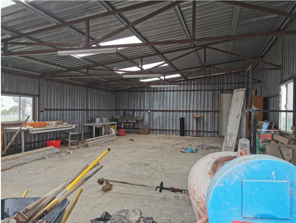
Plate 2 – Internal view of the existing shed subject to alterations and additions
