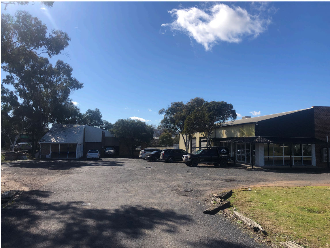
Figure 5 - Photo of existing Unit 9, No. 21 Sydney Road and adjacent building to be demolished.
