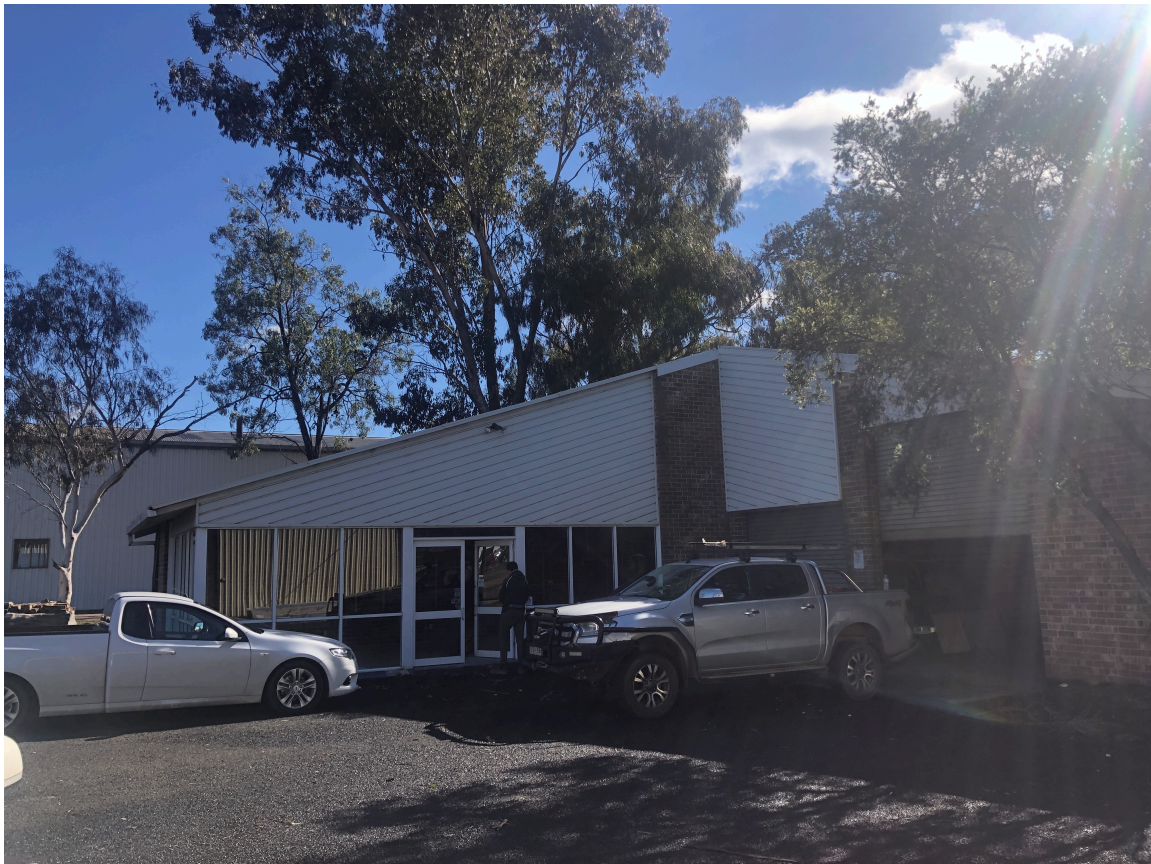
Figure 6 - Photo of existing building to be demolished, No. 21 Sydney Road
