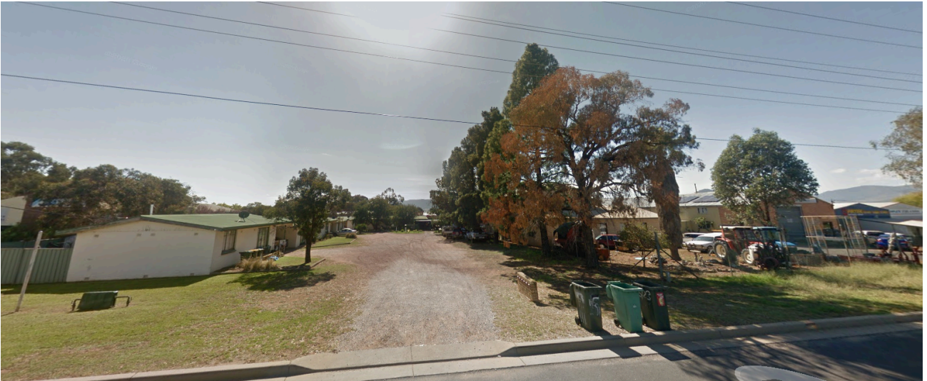
Figure 8 - Photo of existing residential units to be demolished, No. 23 Sydney Road
