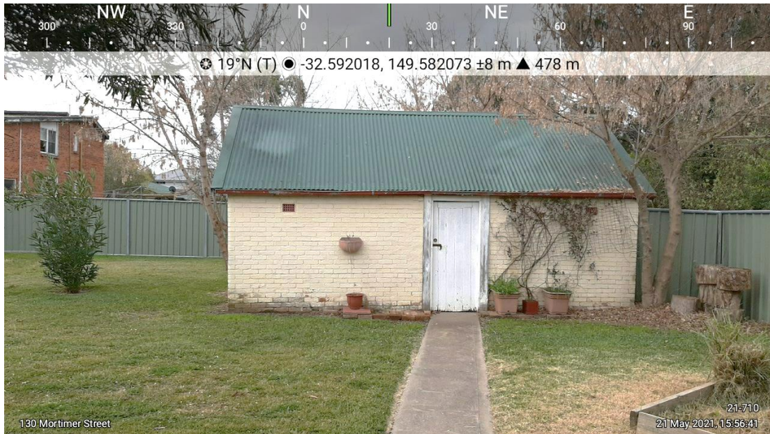
Figure 4 Brick Garage/Shed for Demolition - Side
