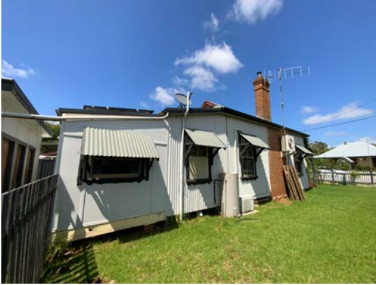
Figure 8: View of the northern elevation facing south.
