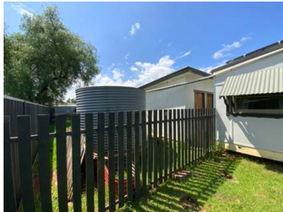
Figure 23: View of the fence separating the front yard from the rear.
