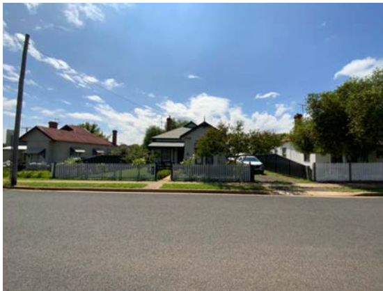
Figure 20: View of the front fence of the site.
