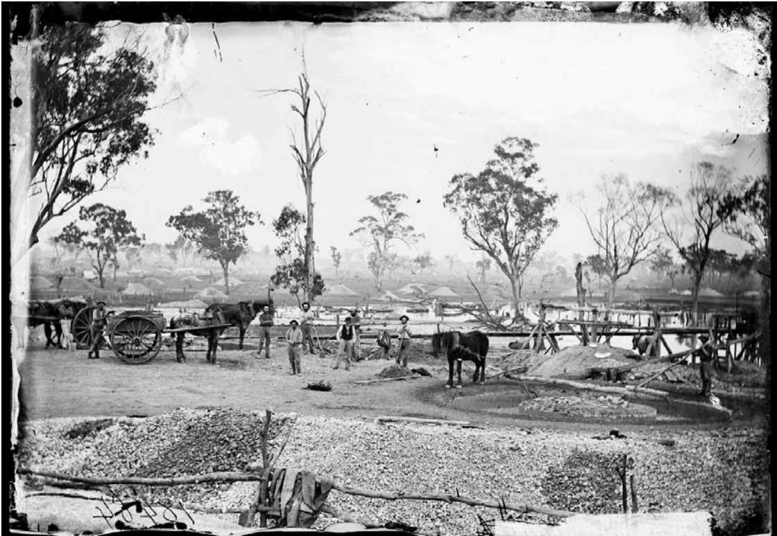
Figure 32: Photograph of the pudding machines in Gulgong during the gold rush, c.1870.
