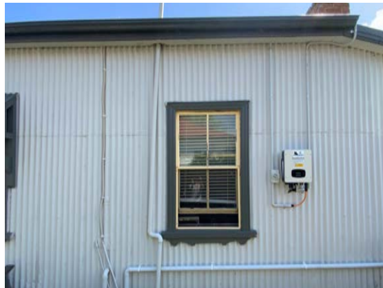
Figure 11: Detailed view of window on southern elevation.
