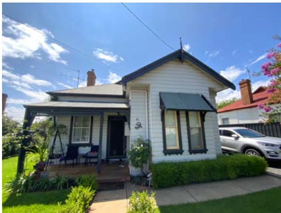
Figure 4: View of the front elevation facing east.
