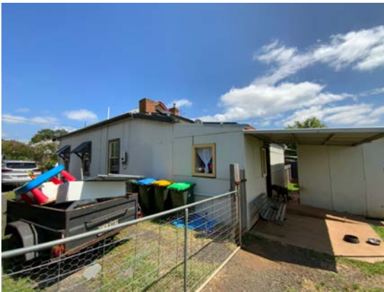
Figure 10: View of the southern elevation facing north.
