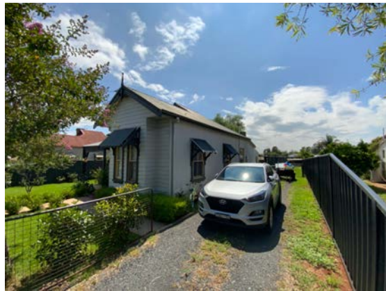
Figure 21: View of the southern driveway and parking area.
