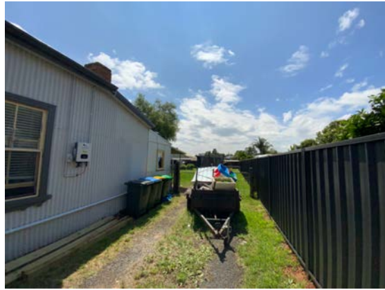
Figure 25: View of the parking space on the southern elevation.
