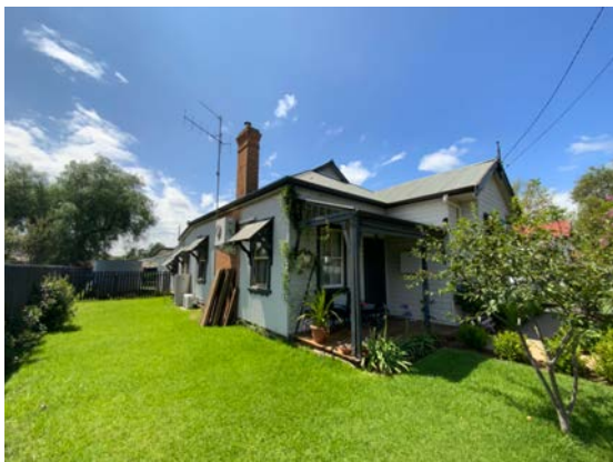
Figure 6: View of the front and north elevations facing southeast.
