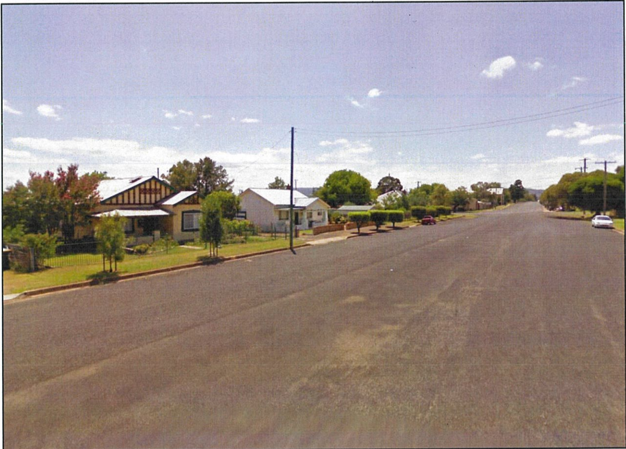
EASTERN VIEW ALONG INGLIS STREET, EXISTING DWELLING ON SUBJECT SITE SHOWN LEFT IN PHOTOGRAPH
