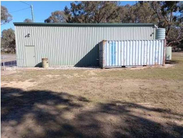
RFS Proposed Site of Extension North Side Looking South
