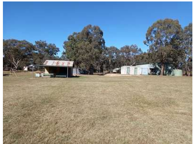
RFS Extension West Side & Facilities Looking East
