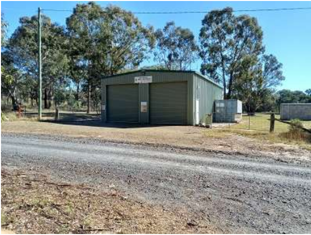
RFS Extension East Side Looking West – Front of Station
