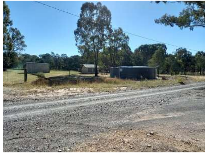
RFS Extension Facilities & Large Tank
