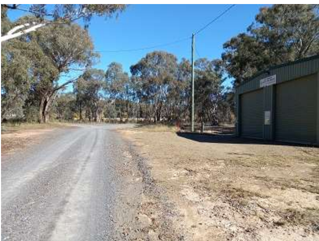
RFS Extension Gardner Street Side - Distance to corner
