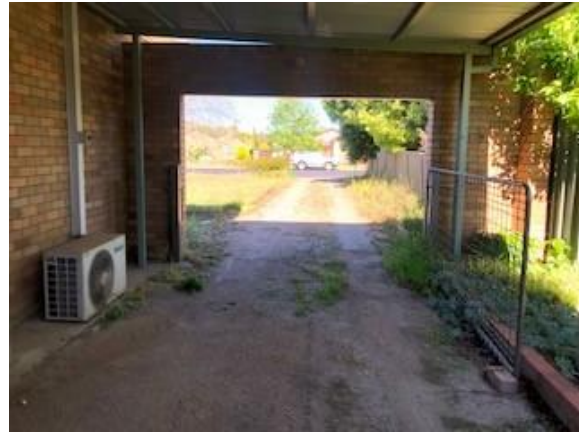
Photo 4: View from within the site, looking east towards George Street
