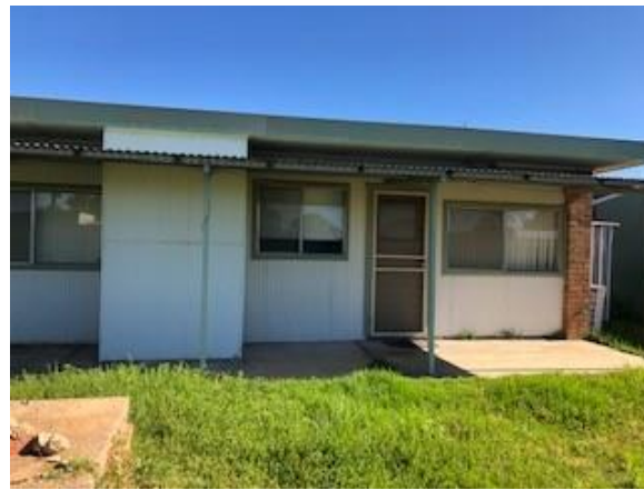
Photo 6: Ancillary structure on site
