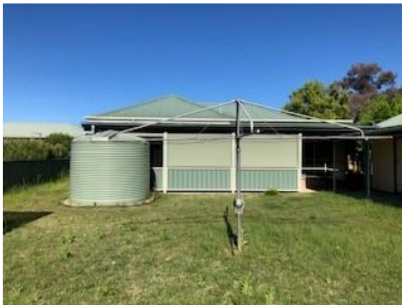
Photo 5: Rear façade of existing dwelling – 46 George Street Mudgee
