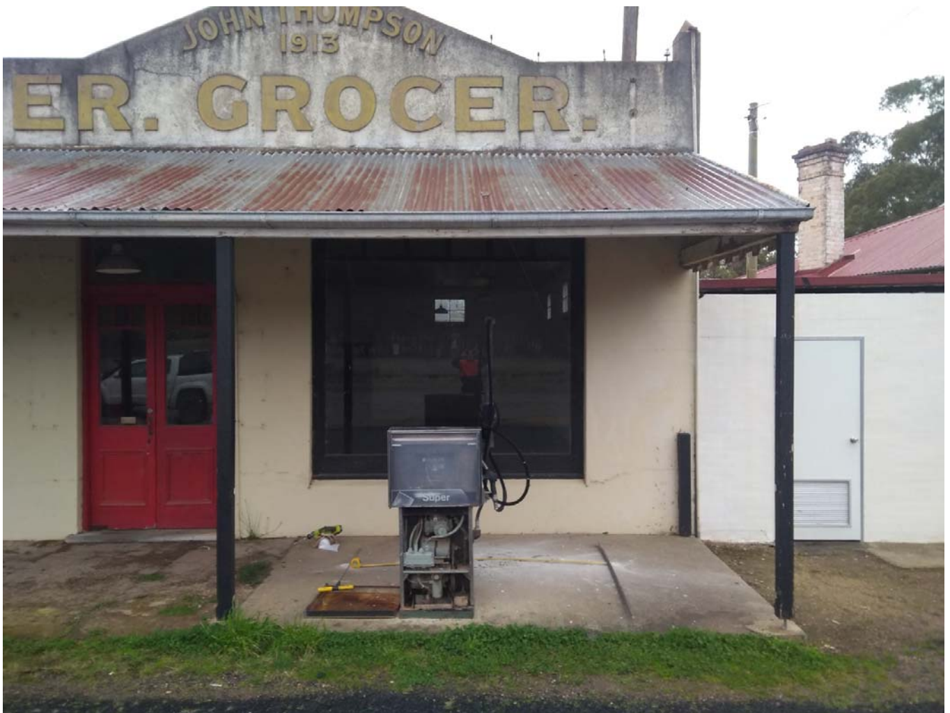
Photograph showing the UPSS area. The pump / dispenser is situated in the foreground. The UST is situated directly beneath the tape measure (beneath the concrete slab). The extended tape measure shows the length of the tank relative to the building and attached awning. The vent riser is the steel pipe mounted to the right (southern) side of the building façade. The concrete slab in the UPSS area appears to be more recent than concrete further to the north (left in this photo).
