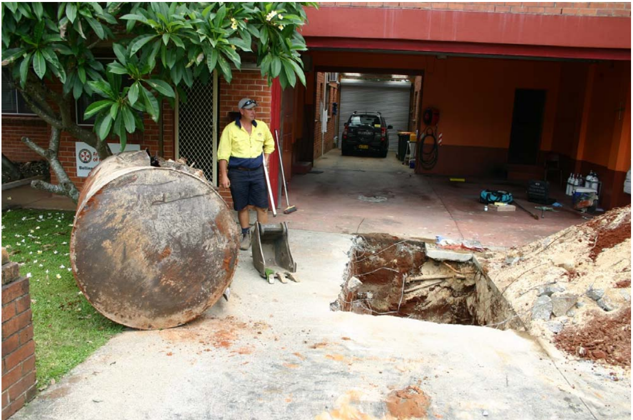
The excavation required to remove the tank only has to be marginally bigger than the tank footprint. This photo shows the extent of excavation to remove the tank and surrounding backfill sand to allow validation sampling of surrounding and underlying soil.
