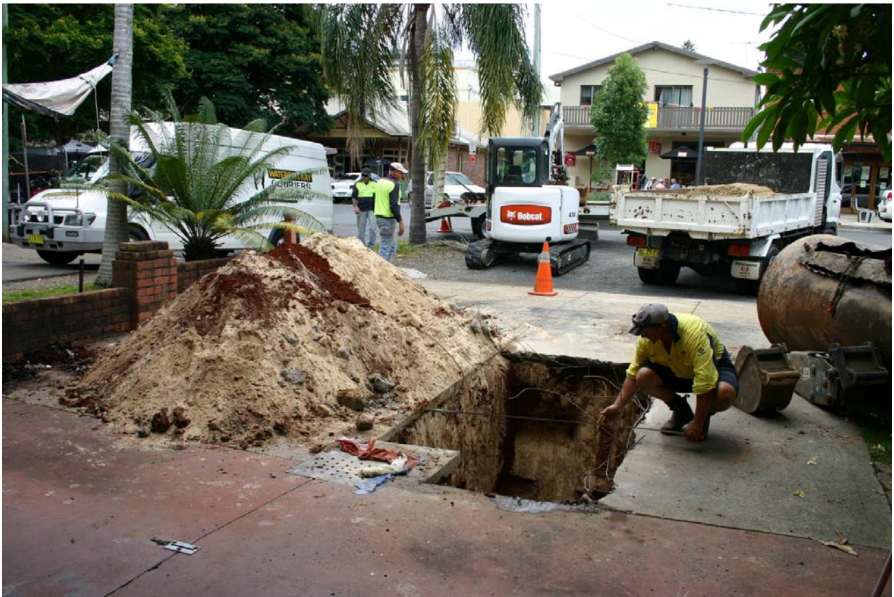
The excavation required to remove the tank only has to be marginally bigger than the tank footprint. This photo shows the extent of excavation to remove the tank and surrounding backfill sand to allow validation sampling of surrounding and underlying soil.
