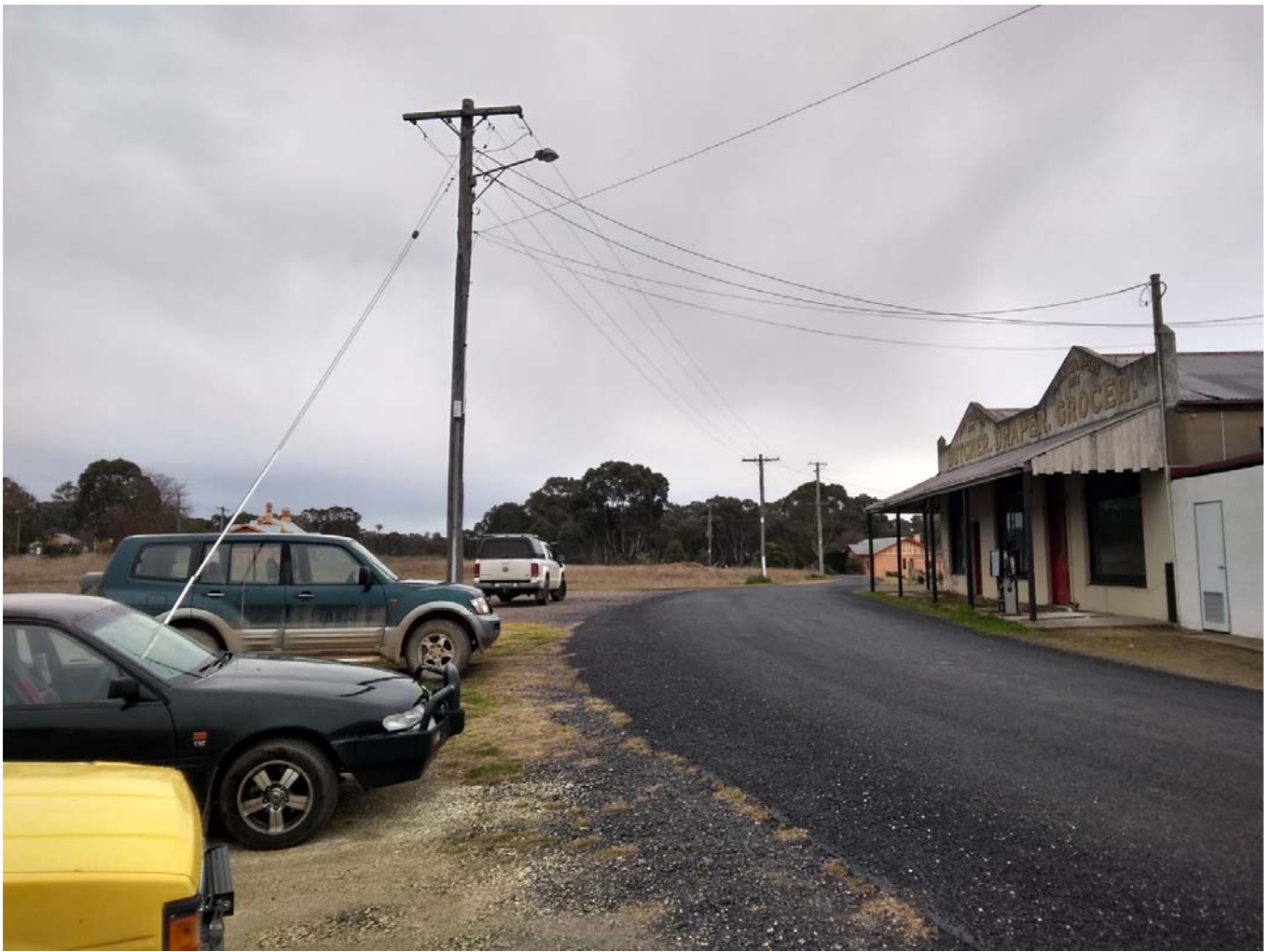
Photo showing surrounding area. Machinery will have to be positioned on the road during the works. We will implement a traffic control plan for the works.
