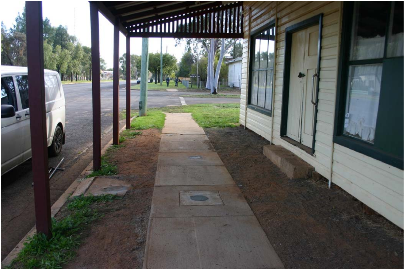
In 2016 Ground Doctor and AWF removed a UPSS from an old general store at Baradine, NSW. The UPSS was situated in the footpath beneath the awning of an adjacent building. The UPSS was comprised of 3 tanks including two 2200L tanks and one 4500L tank.
