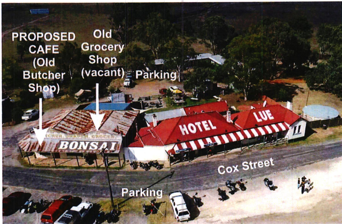
Figure 1. Showing the Lue Hotel (right) and Thomson building (left). Looking north.
