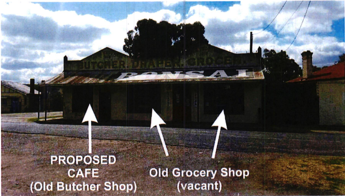
Figure 2. Thomson building. Looking north.
