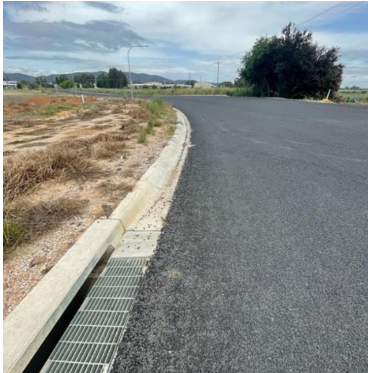
Plate 2 – View of kerb and guttering on Burrundulla Road, sealed
