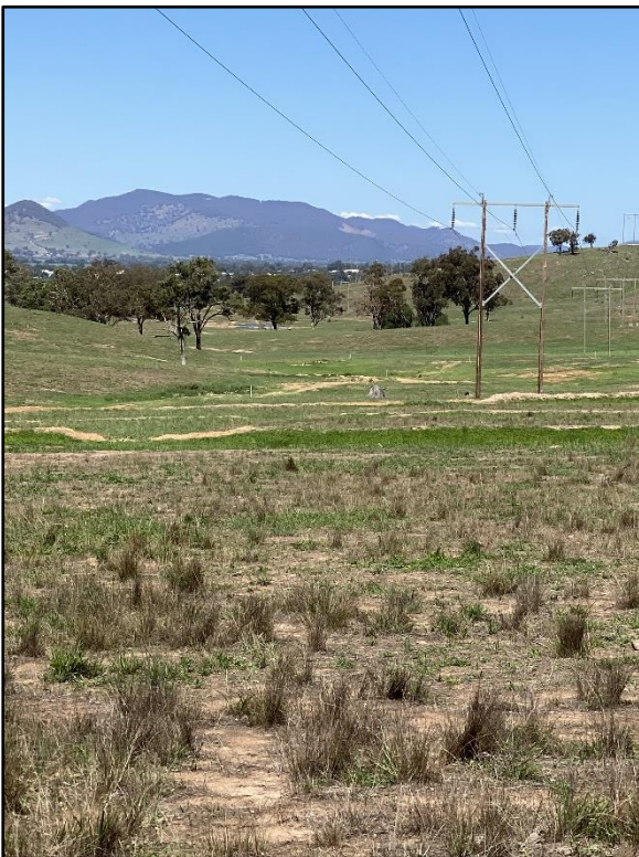
Plate 7: View to east along location of most northern first order mapped drainage line originating from STP infrastructure (partly constructed diversion bank) within Lot 289
