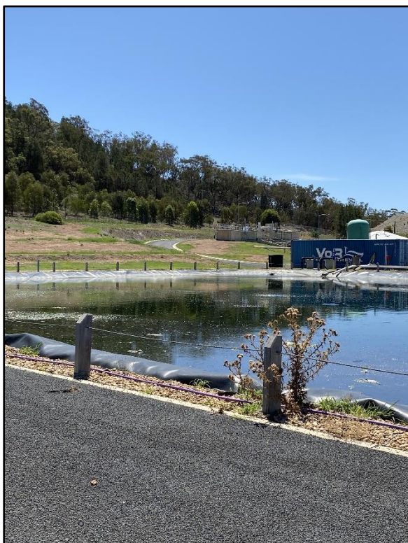
Plate 3: View to north-west from closest sewage pond to the proposed site (access road to be extended).
