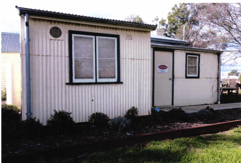
Figure 4 Rear view of house showing bathroom and extended verandah.
