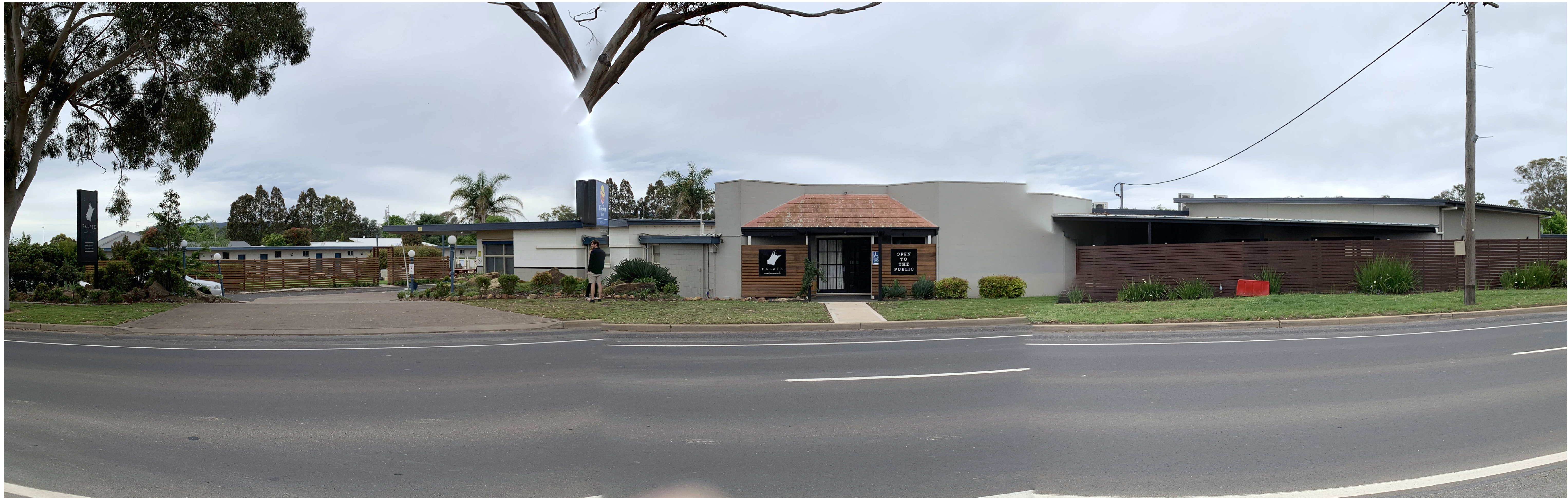
EXISTING STREETSCAPE SHOWING MAIN ENTRY, RECEPTION, RESTAURANT AND FUNCTIONS (PHOTO STITCH)
