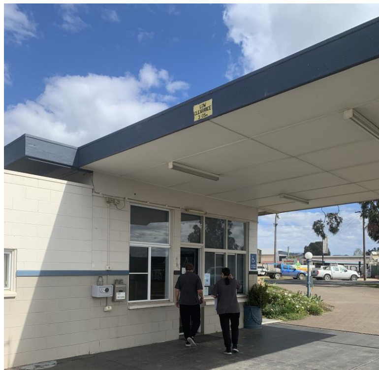
Plate 3 – View of the current reception area to be improved
