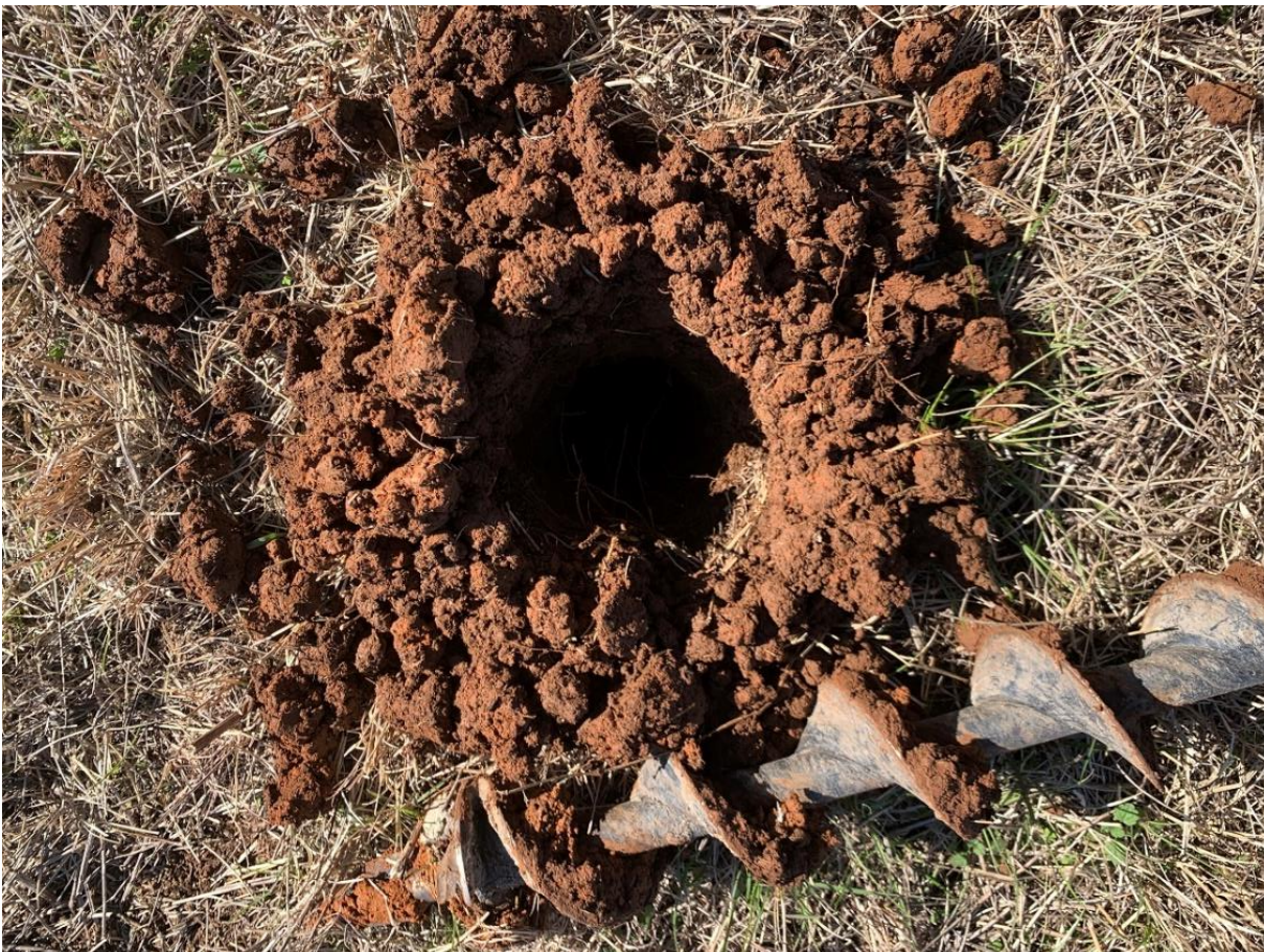
Figure 3: Borehole 1, excavated onsite.
