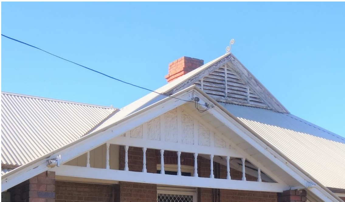
Figure 9 Decorative gables and wrought iron finial.
