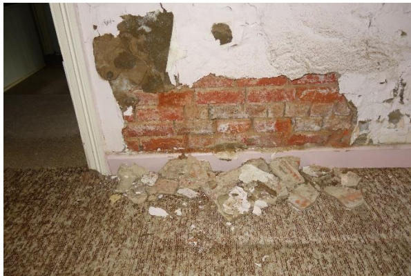
Figure 7: Sections of damp walls in the Federation section of the house.
