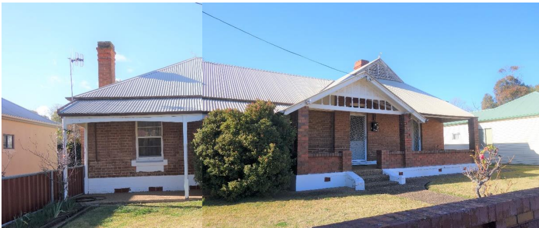
Figure 4: Existing Street façade.
