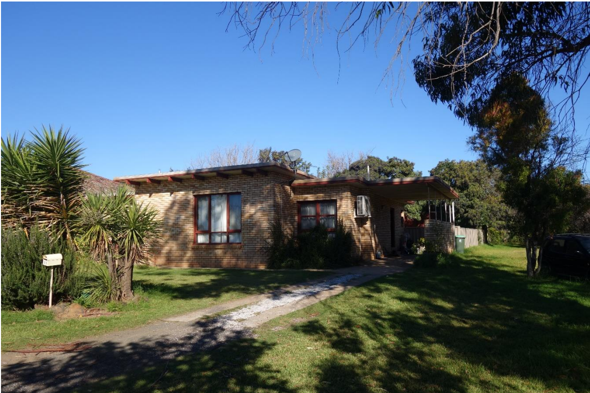
Figure 1: Front view of Residence proposed to be demolished.
