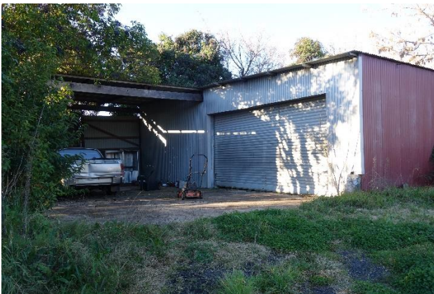
Figure 4: rear shed on laneway.
