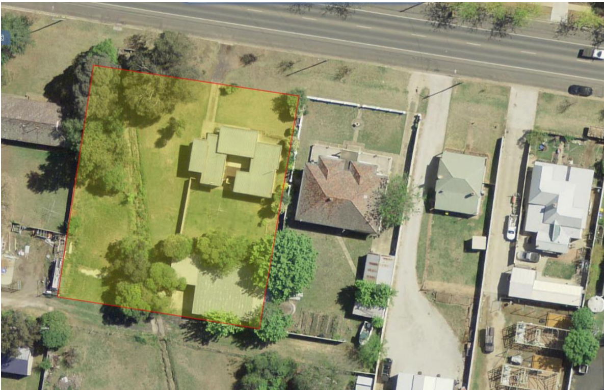
Figure 2 Aerial view from Six Maps. The house and shed behind it, are proposed to be demolished.
