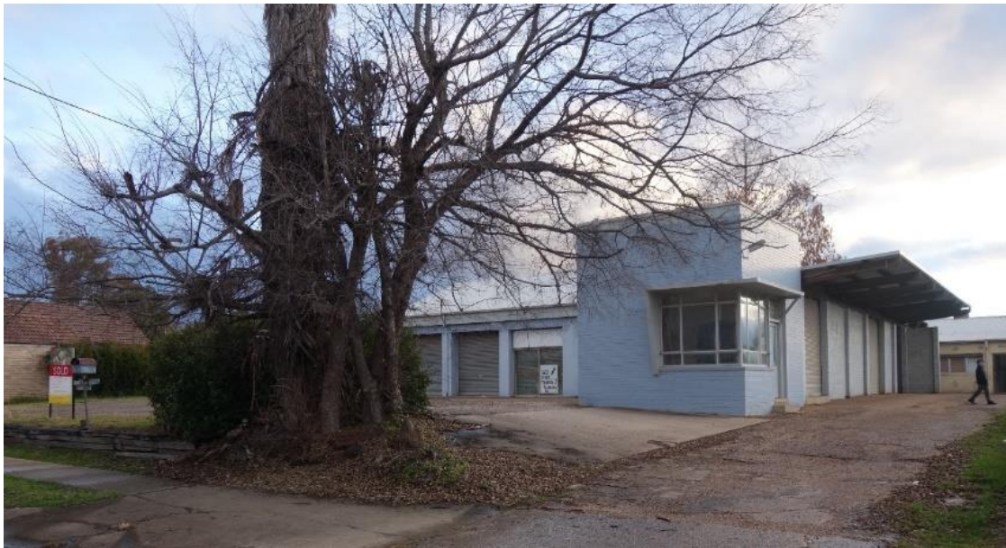
Figure 8 Front view showing office space added c. 1970s
