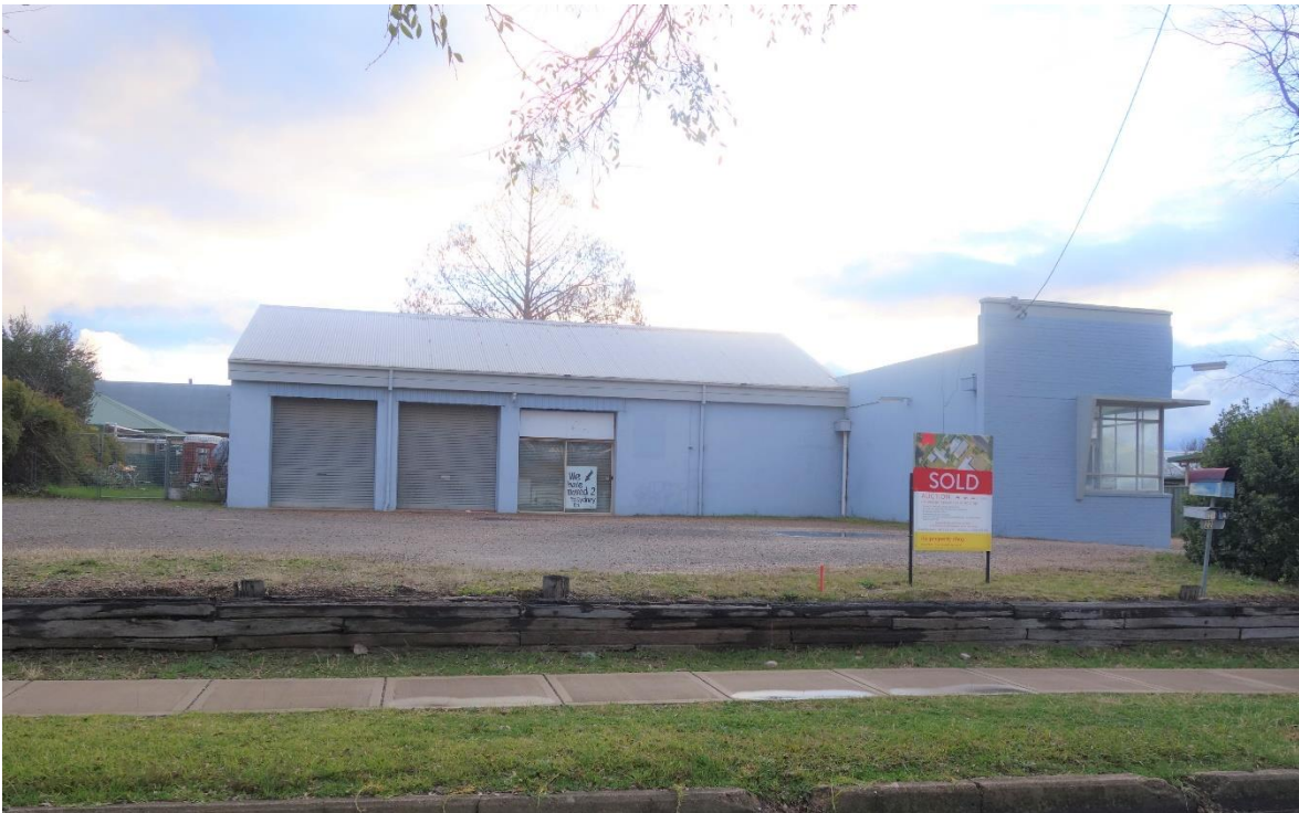
Figure 1: Front view of industrial buildings proposed to be demolished.
