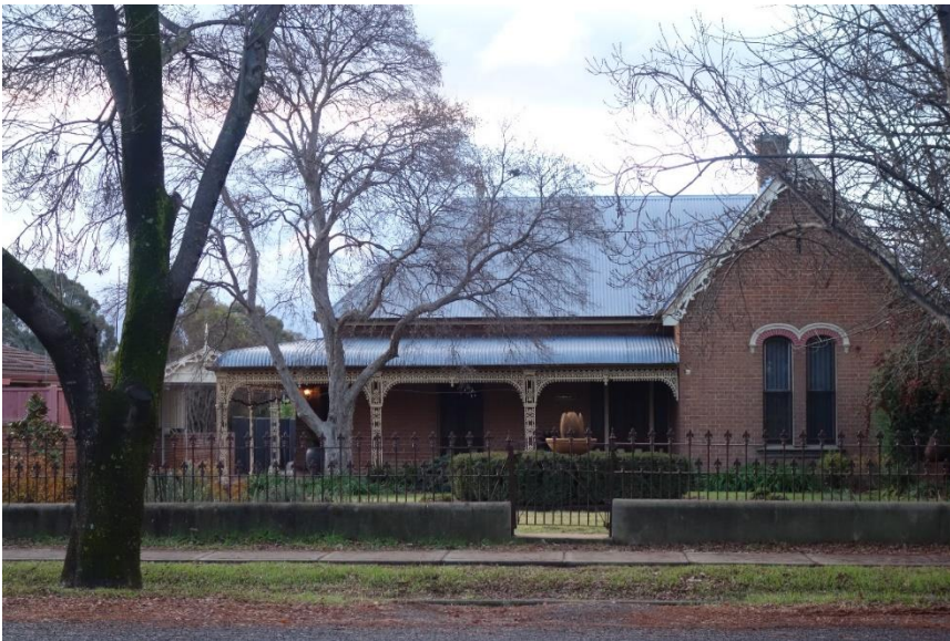
Figure 4 Heritage item I 151 at 64 Mortimer Street Mudgee. Façade facing Mortimer Streetscape.
