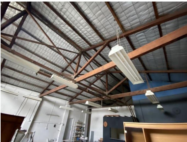
Figure 10 internal roof trusses
