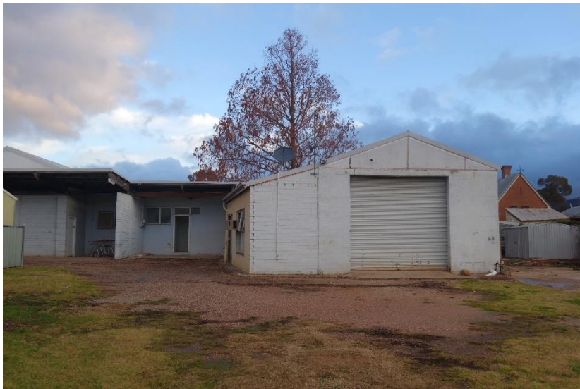
Figure 14 some of the small sheds on the site
