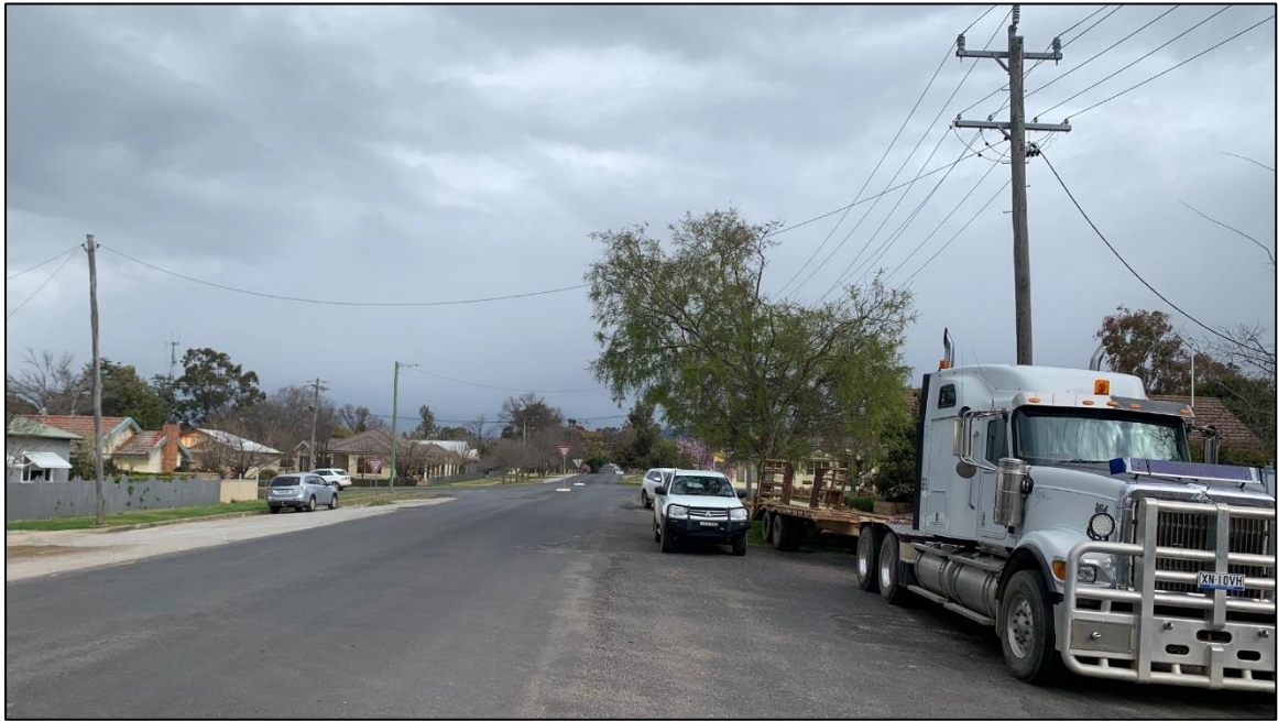
Plate 1 – Looking South along Lawson Street from the front of the site
