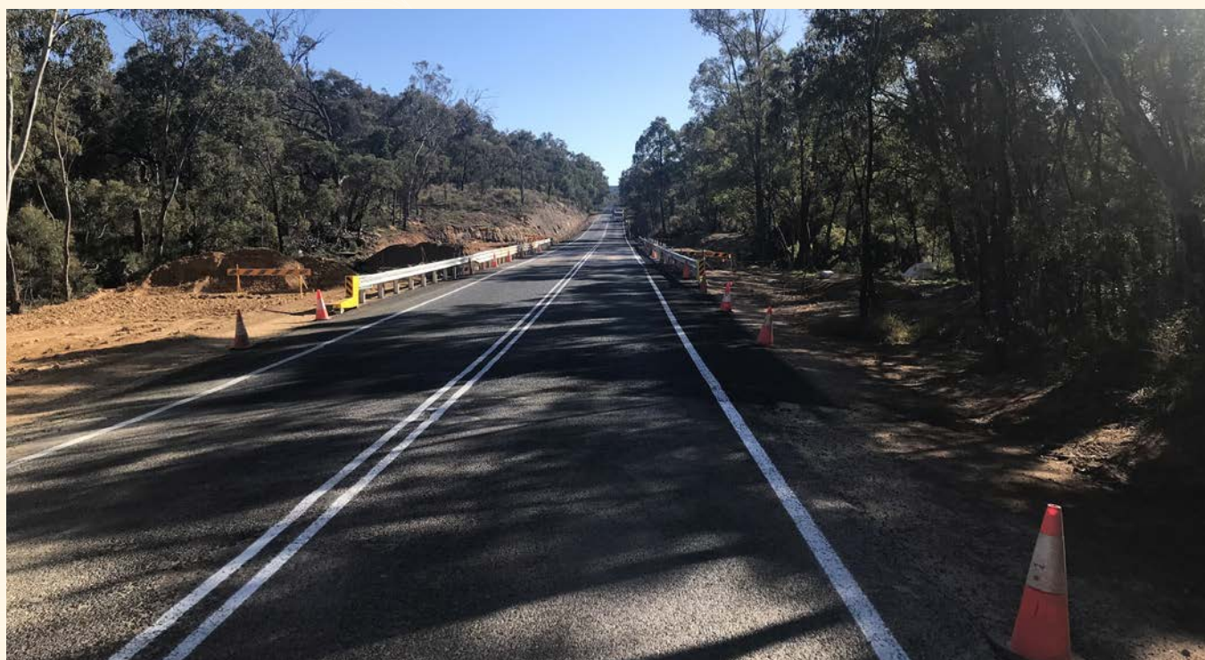
> Goulburn River Bridge replacement
