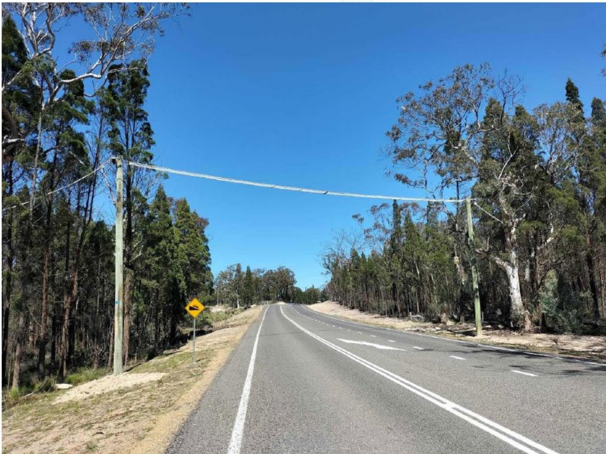
> Aerial fauna crossing, Wollar Road
