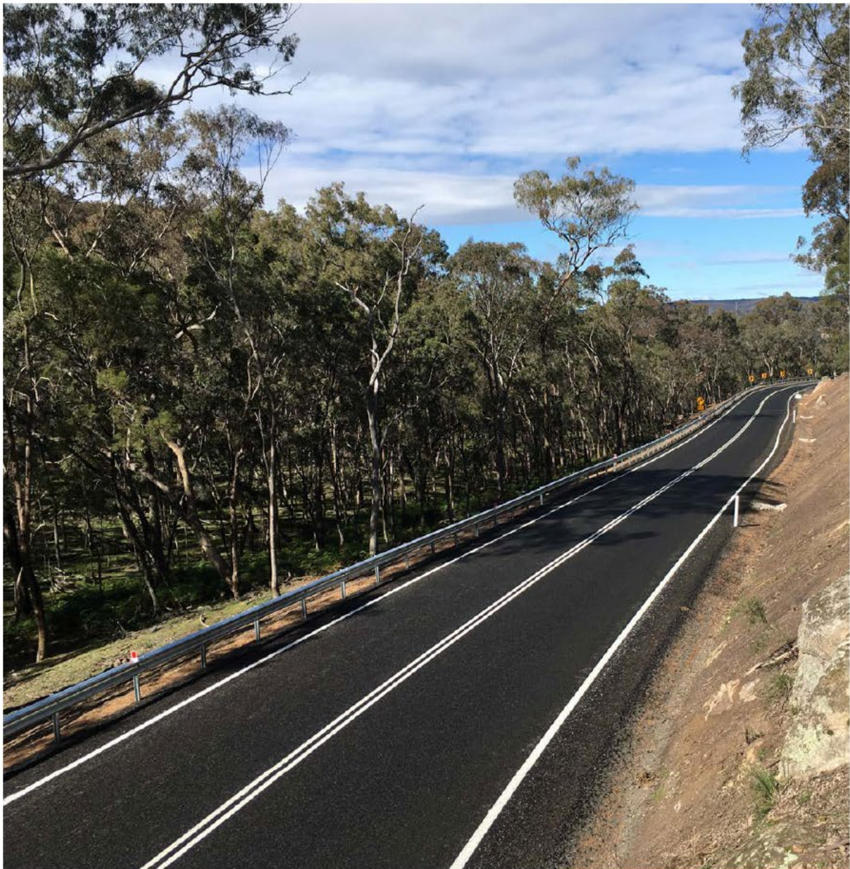
> Wollar Road Upgrade
