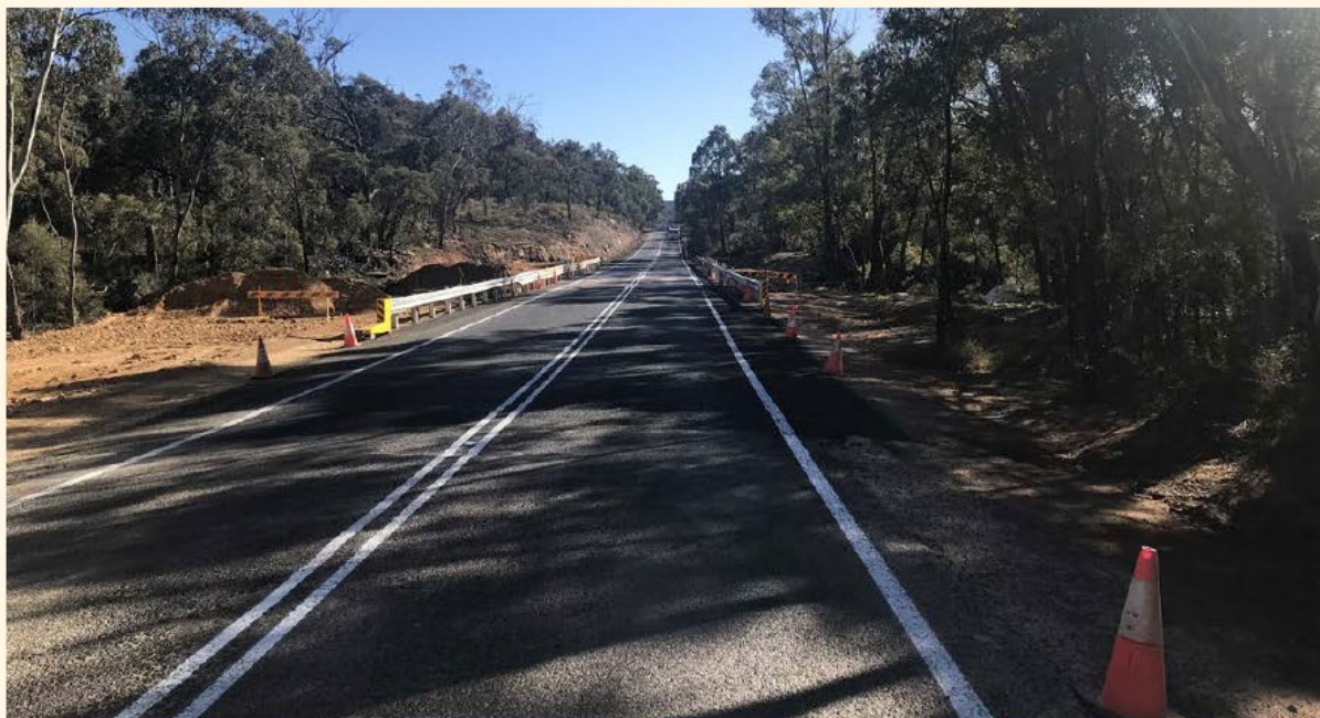
> Goulburn River Bridge replacement
