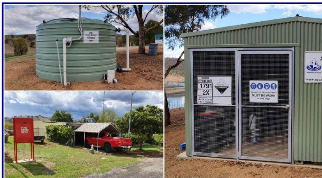
Figure 19 – Assets Holiday Park: Water Infrastructure Top LHS clockwise: Water treatment plant; fire hydrant.
