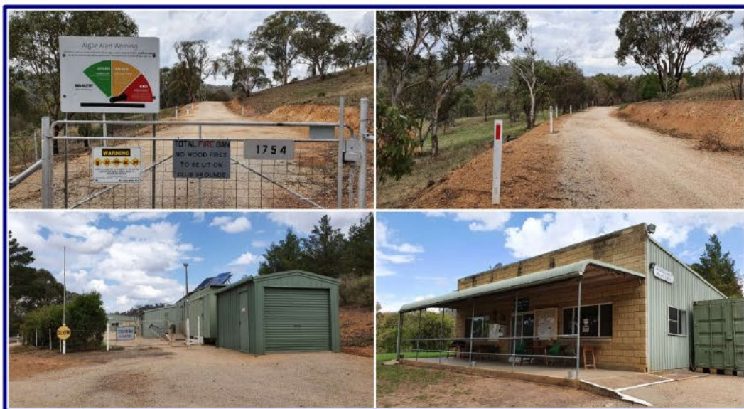
Figure 21 – Assets Anglers Club Top LHS clockwise: Entrance gate and signage; all-weather access road; Clubhouse; Amenities/sheds. Lot 3.
