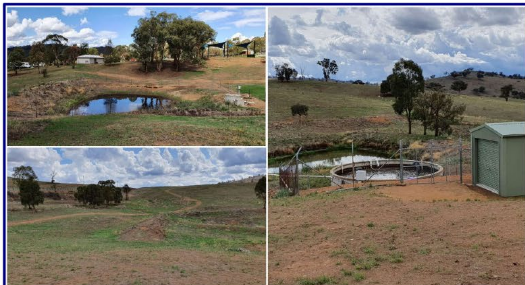
Figure 8 – Topography, Hydrology and Drainage Diversion banks and small dams used for runoff management and supplying essential services at Cudgegong Waters Park.
