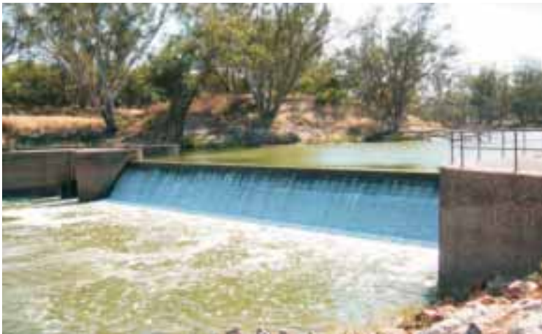
ABOVE Bourke Weir.
