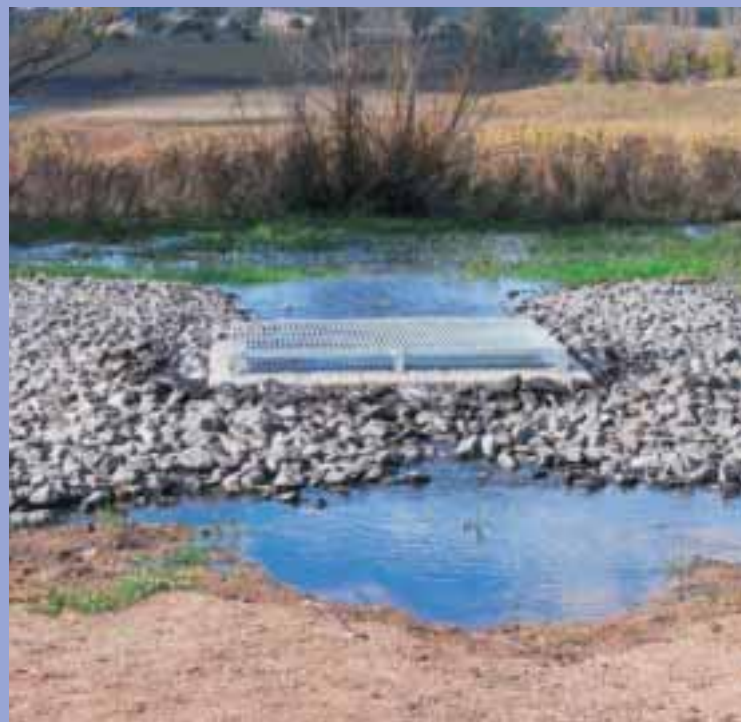
Harvested stormwater entering Suma Park Dam, Orange.
