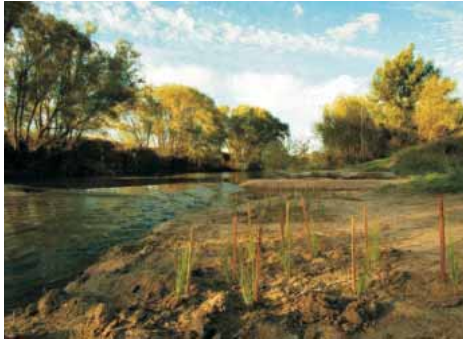
ABOVE Re-vegetation works, Macquarie River, Bathurst (source: David McKellar).
