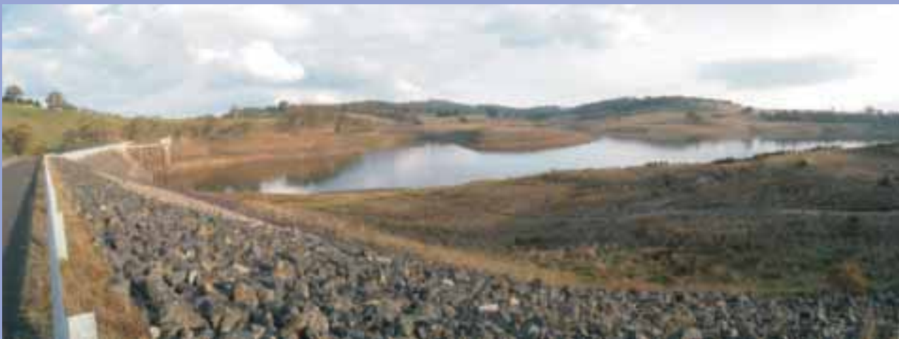
Oberon Dam in May 2009 at 12.5% capacity
