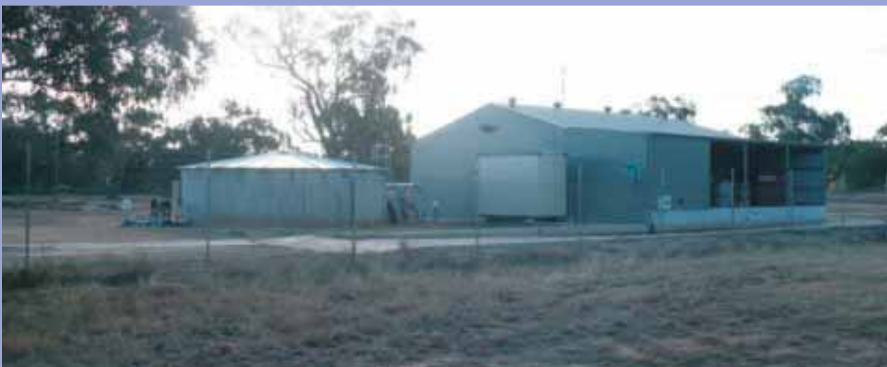
Mendooran drinking water supply facilities on the Castlereagh River
