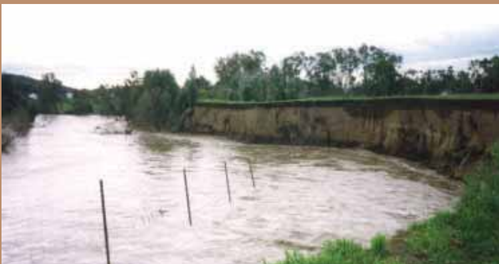
Riverbank erosion on the Bell River, Wellington.
